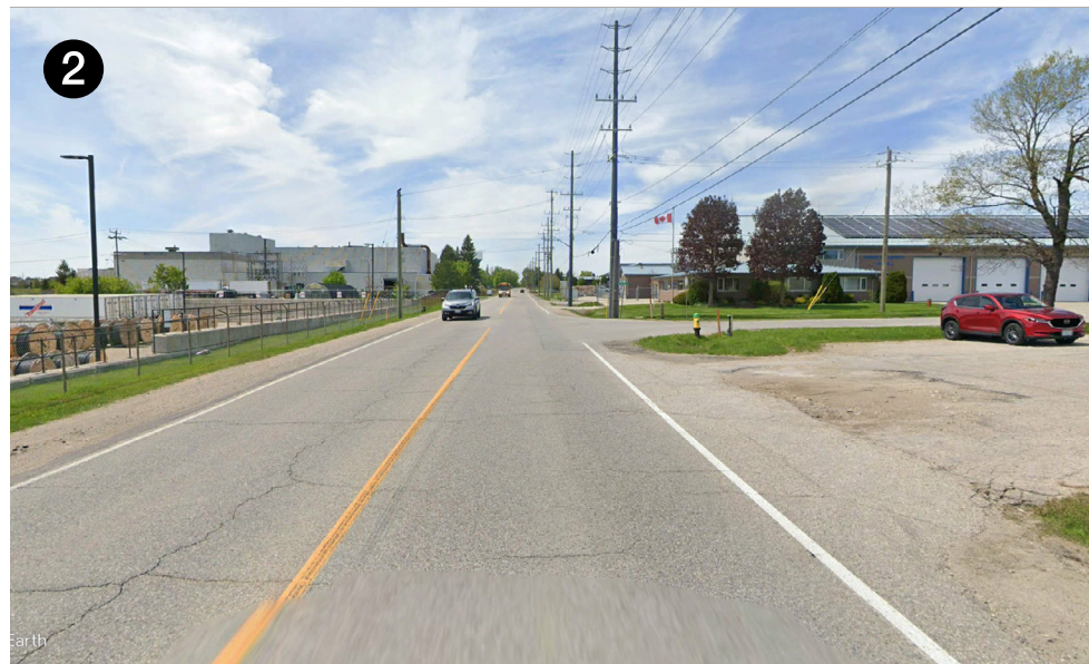
View along Garthshore St, Facing Northwest, Employment Uses
