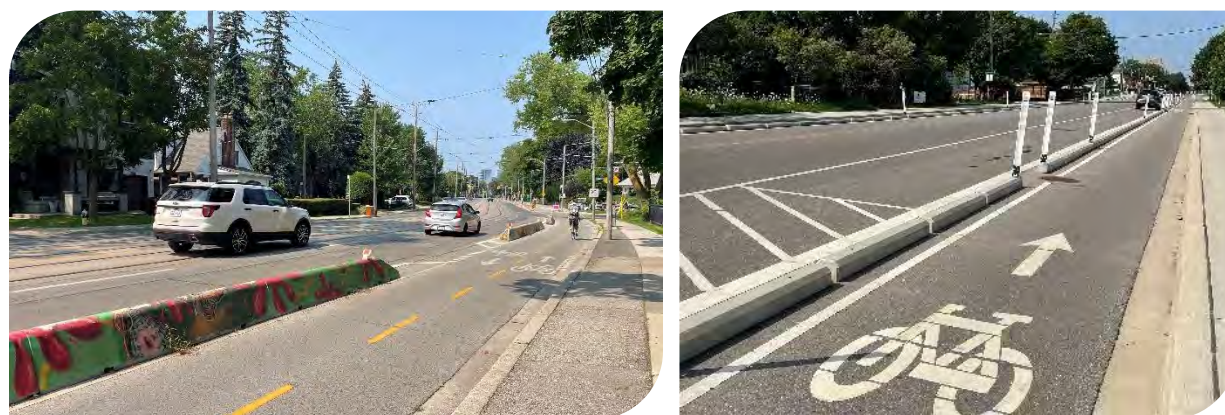
Figure 5.8: Examples of protected bike lanes in Toronto. Separation techniques include concrete barriers with public art (left) and Concrete curbs with flex posts (right).
