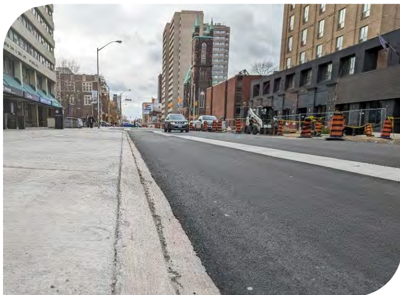
Figure 6.2: Example of a bevelled curb between a cycle track and sidewalk, Toronto
