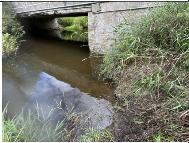
Photo 8: Erosion on the downstream's east bank, small patches were present on the west as well. Facing west.
