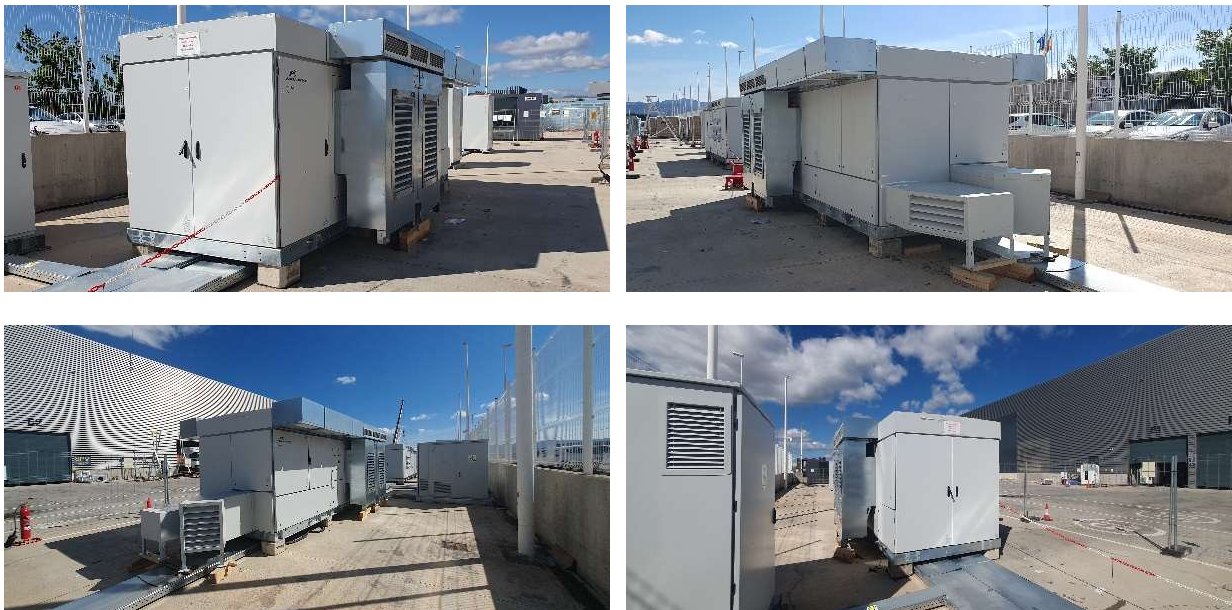
Illustration 2. PCSM Gen3 Inverter with acoustic attenuation kit
