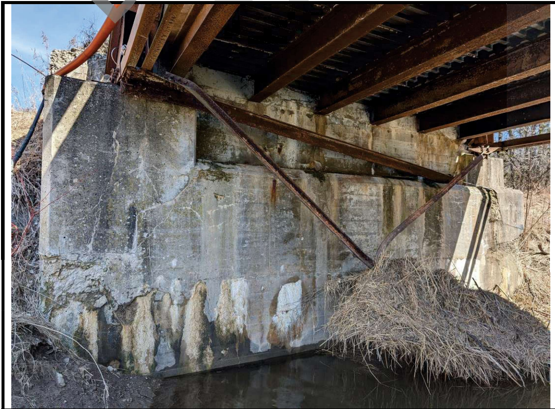
Photo 12 Damaged bracing at east end of structure
