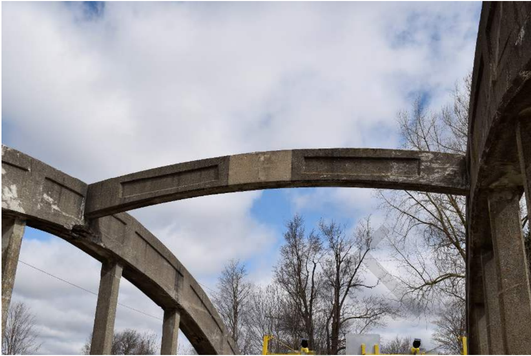
Figure 34: Original cast concrete tie beam
