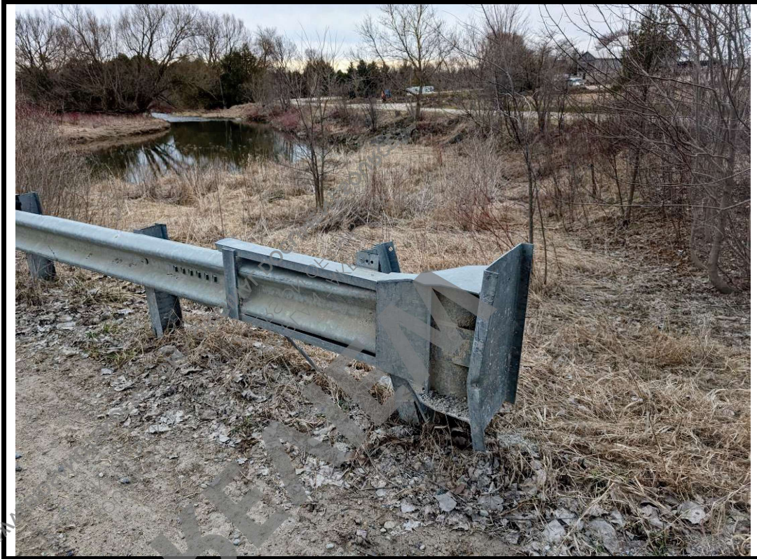
Photo 7 Vehicle damage on northeast end treatment
