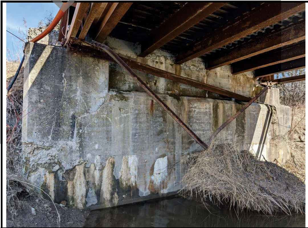
Photo 16 Severe concrete disintegration with area of heavy efflorescence at west abutment.
