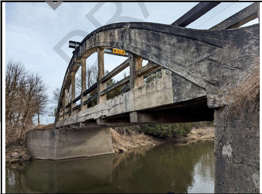
Photo 16 Wide cracks with stains and spall noted on east exterior soffit
