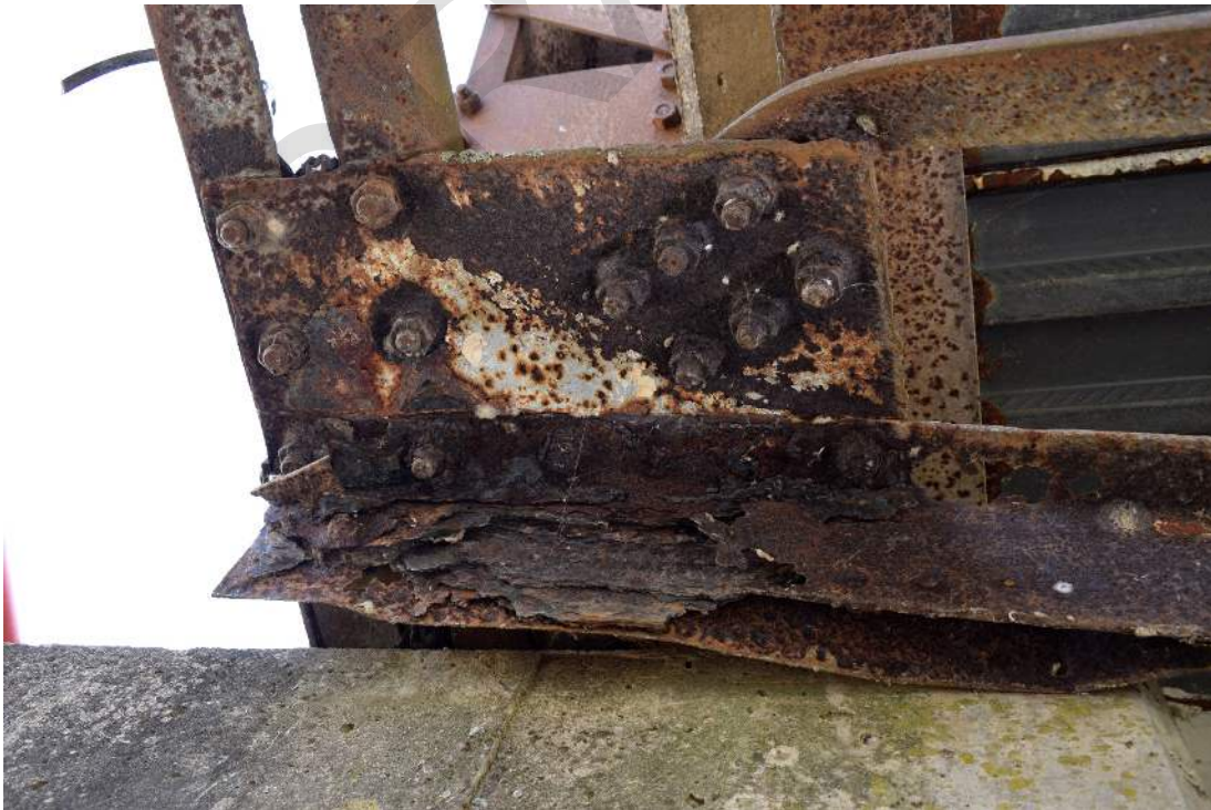
Figure 48: Example of typical deterioration of structural steel
