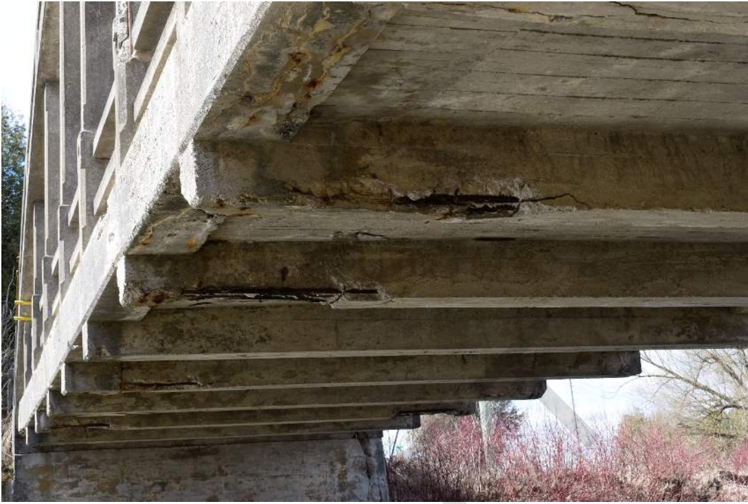
Figure 30: Underside of Bridge 29-WG, note presence of imprints of original wood forms
