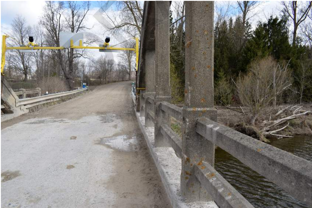
Figure 35: Typical example of the details present in the original guard rail and support structure
