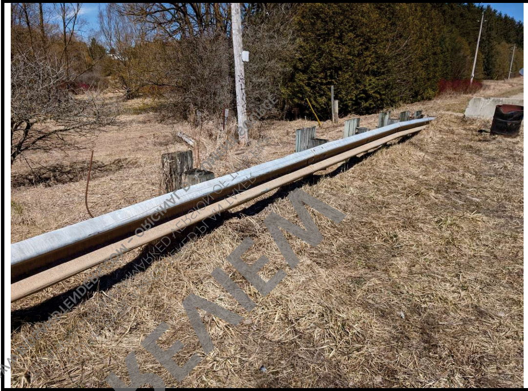
Photo 7 Substandard approach barrier at NE approach
