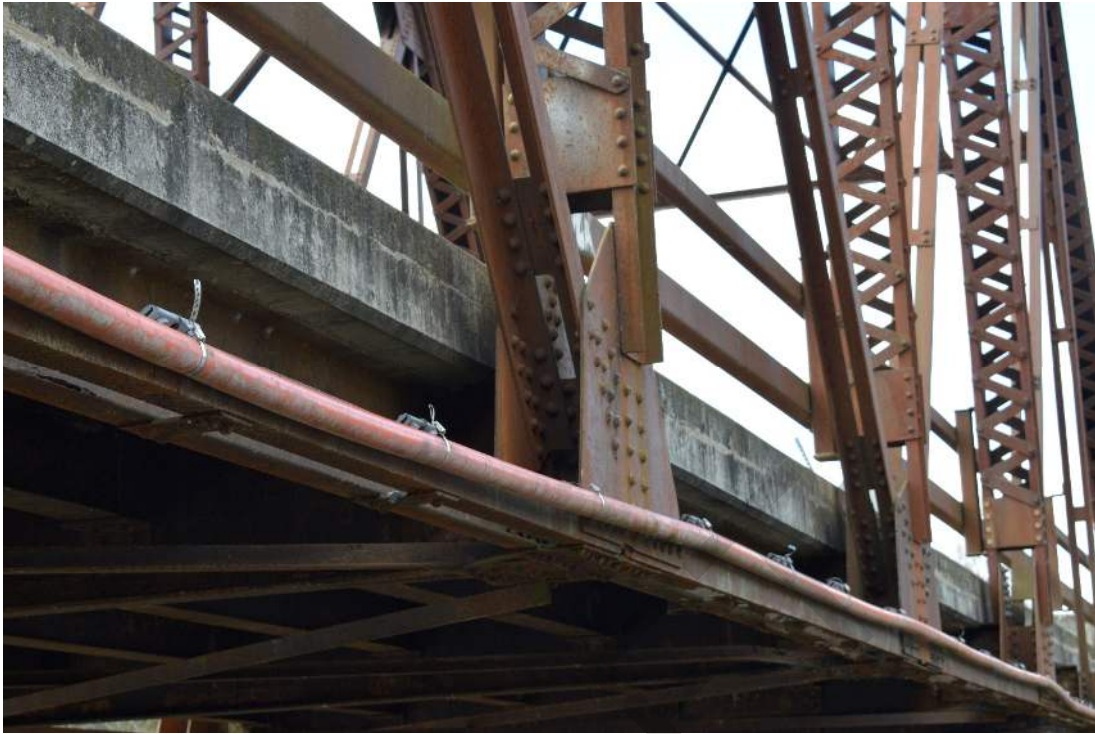
Figure 49: Example of original riveted construction
