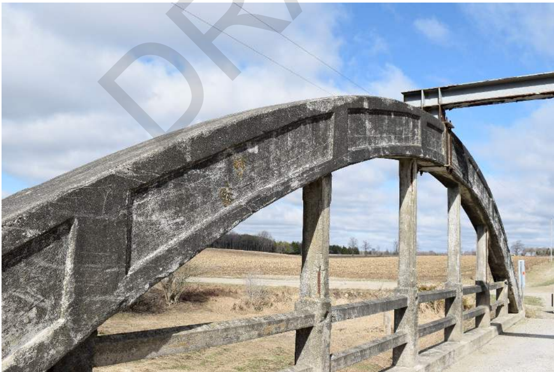
Figure 16: Close up of detail cast into arch and associated supports and guardrail, west side
