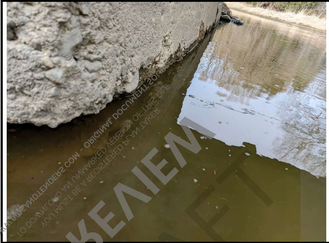
Photo 19 Severe erosion observed at the base of the northwest wingwall.
