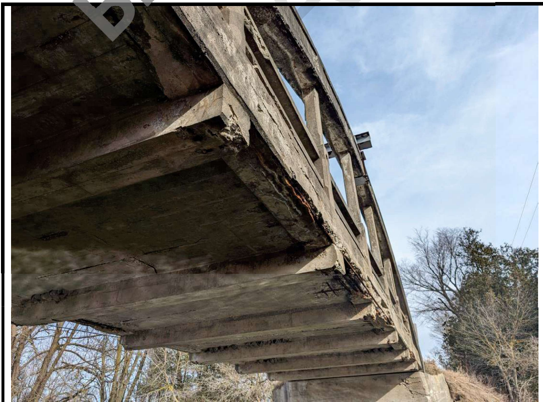
Photo 20 delaminations, narrow cracks with efflorescence and spalls with exposed corroded reinforcement noted at ends of floor beams
