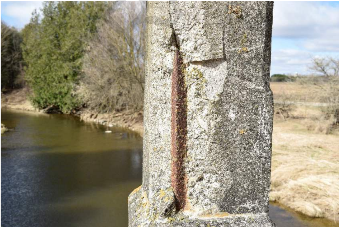
Figure 22: Example of smooth square reinforcement bar used in vertical support members
