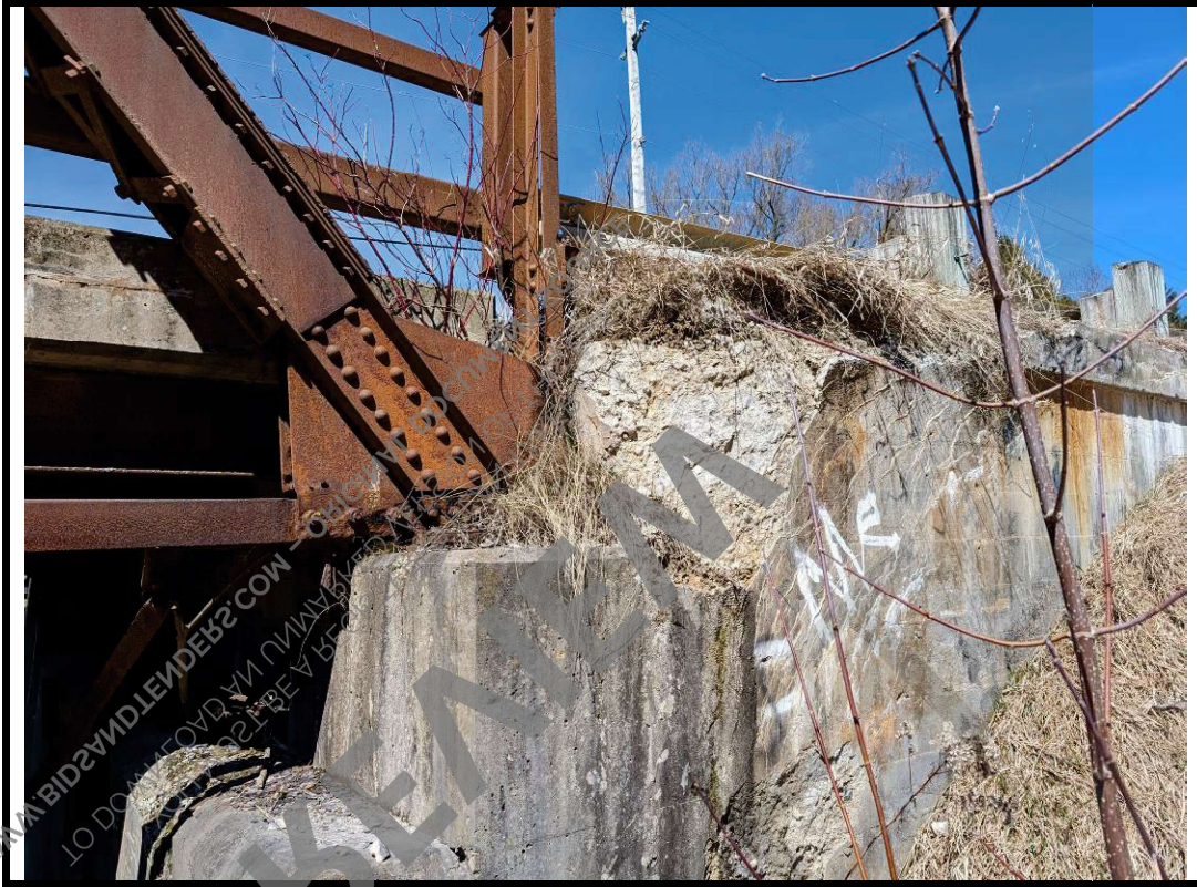
Photo 13 Concrete Disintegration at SE wingwall
