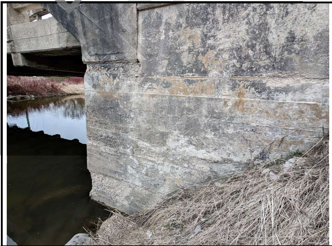
Photo 20 Moderate scaling and severe concrete disintegration southeast wingwall interface
