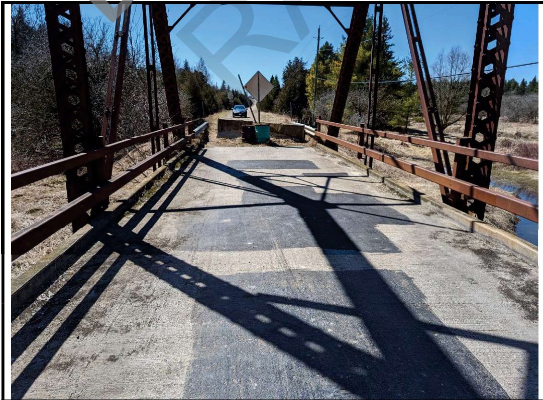
Photo 8 Previous asphalt patches on deck wearing surface
