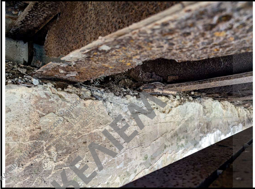
Photo 17 Top of east of ballast wall is completely disintegrated with severe scaling
