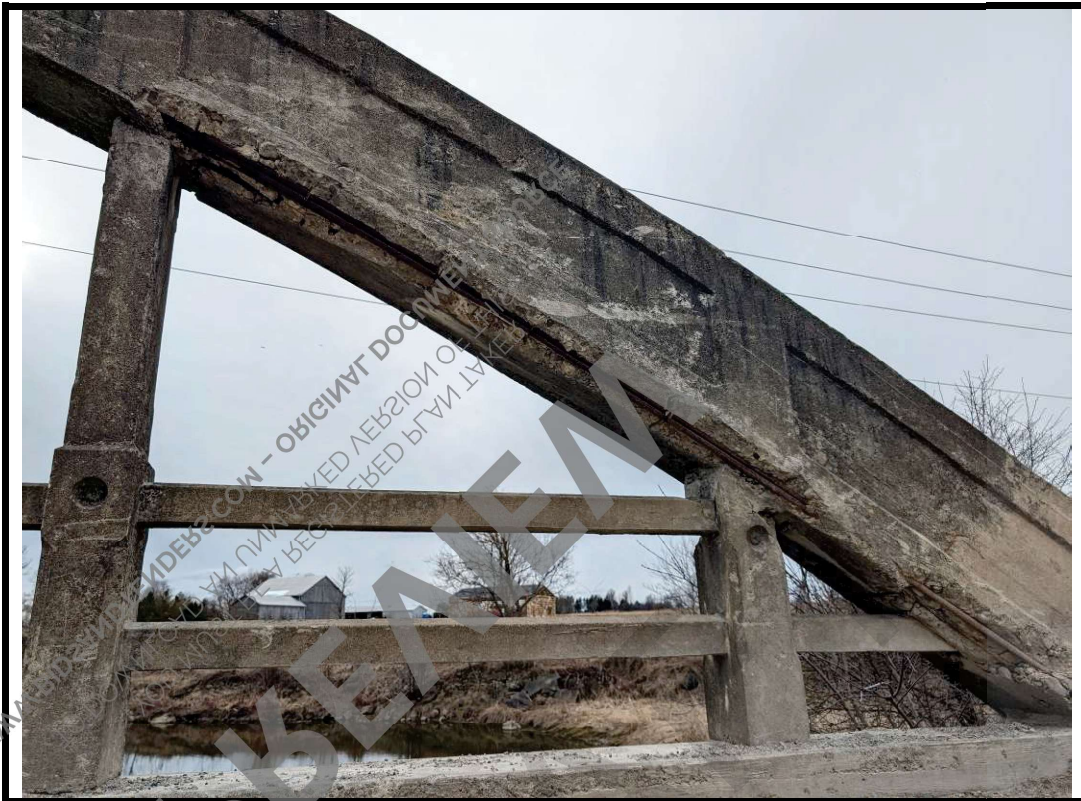
Photo 11 Spall with exposed corroded reinforcement on north truss
