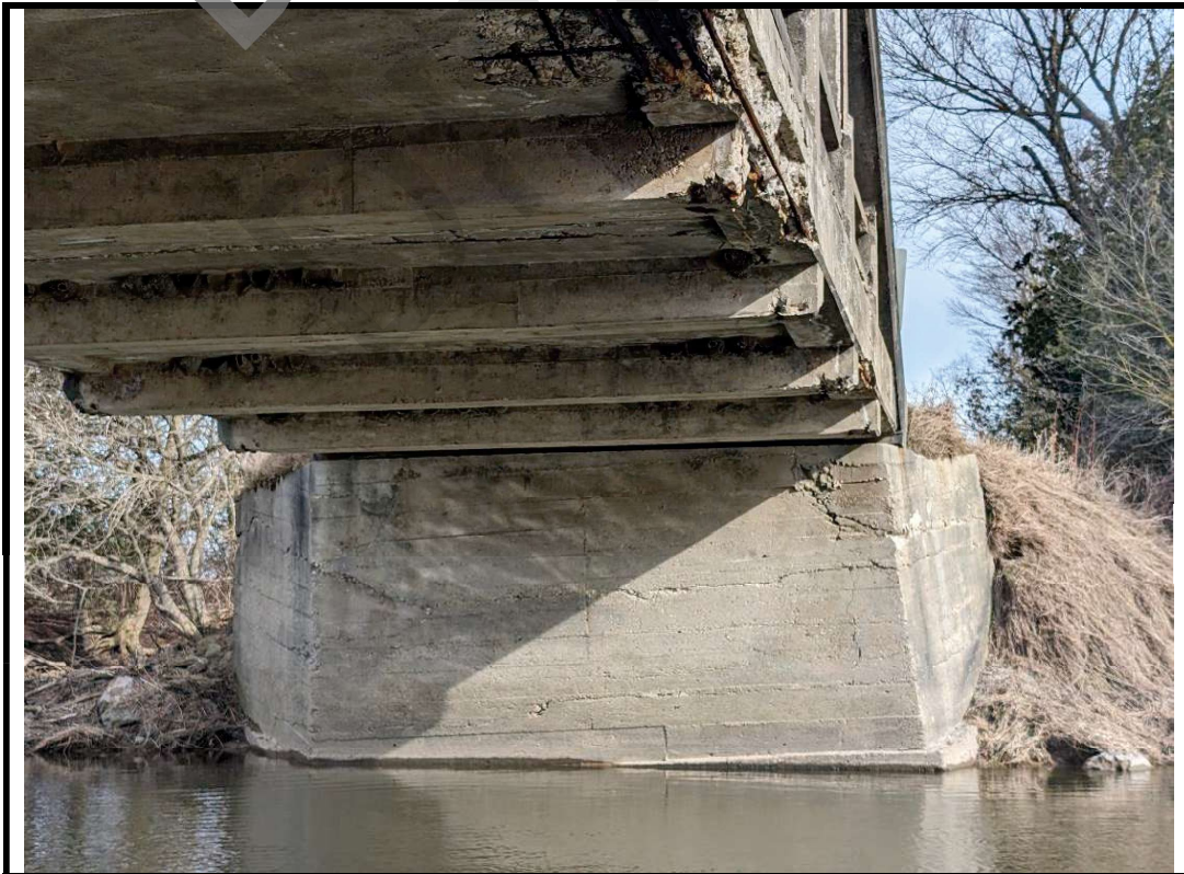
Photo 14 Southeast corner of foundation appears to have settled.
