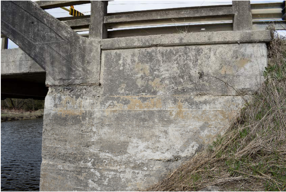
Figure 32: Example of connection between Bridge 29-WG abutments and superstructure
