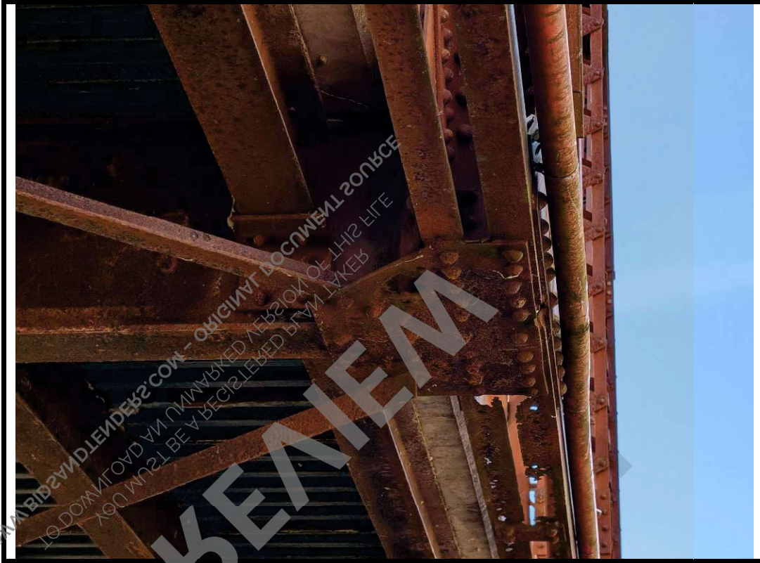
Photo 15 Severe corrosion and section loss at connections in the structure.
