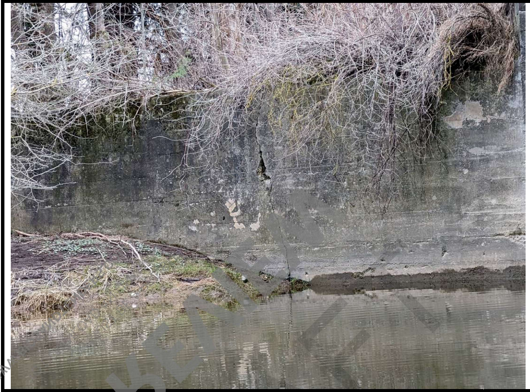
Photo 21 Vertical wide crack on southwest wingwall
