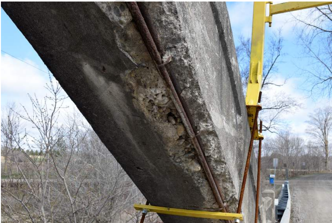
Figure 37: Example of exfoliated concrete exposing underlying smooth steel reinforcement
