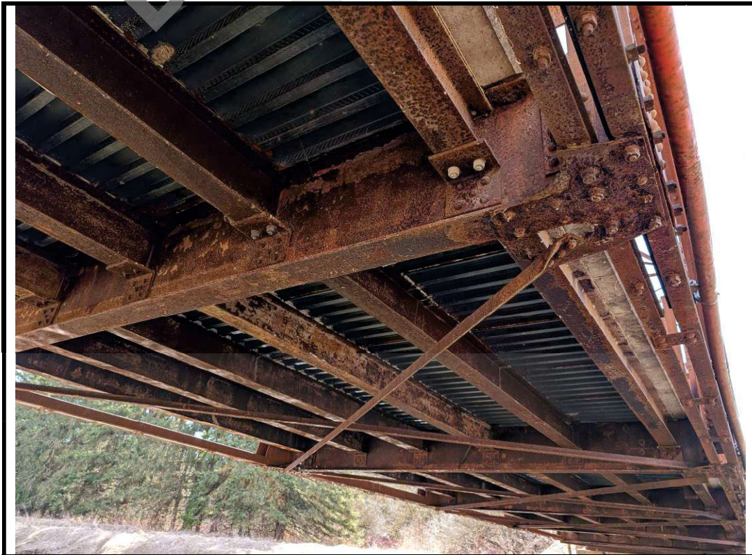
Photo 10 Perforations on north bottom chord
