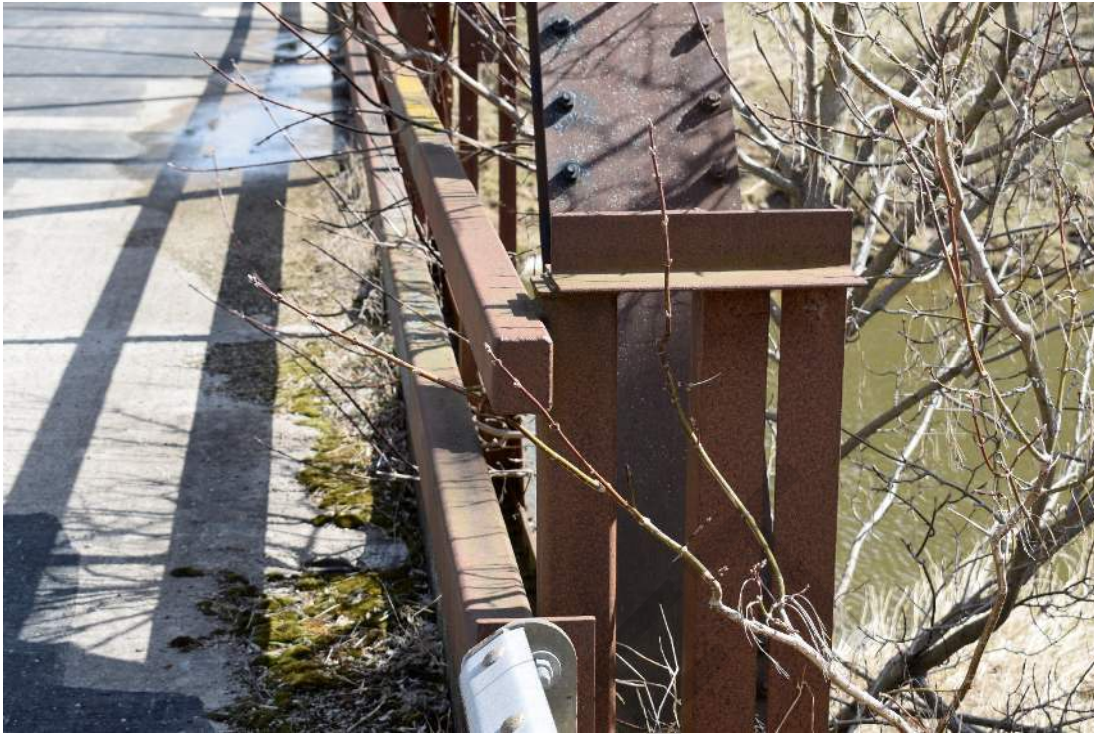
Figure 51: Non-original guard rail installed using modern welding techniques
