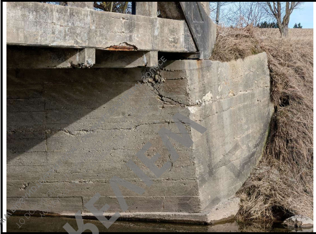
Photo 13 South abutment wall appears to be rotated inwards.
