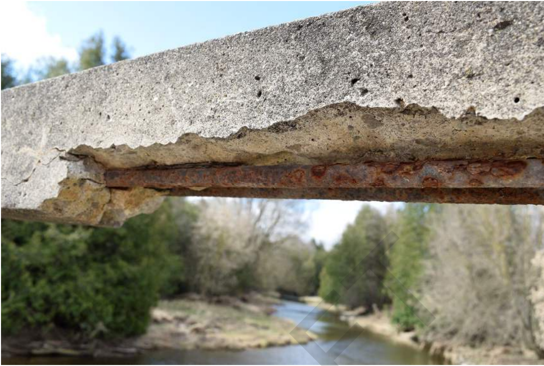
Figure 21: Example of smooth round reinforcement bar used in construction of guardrails
