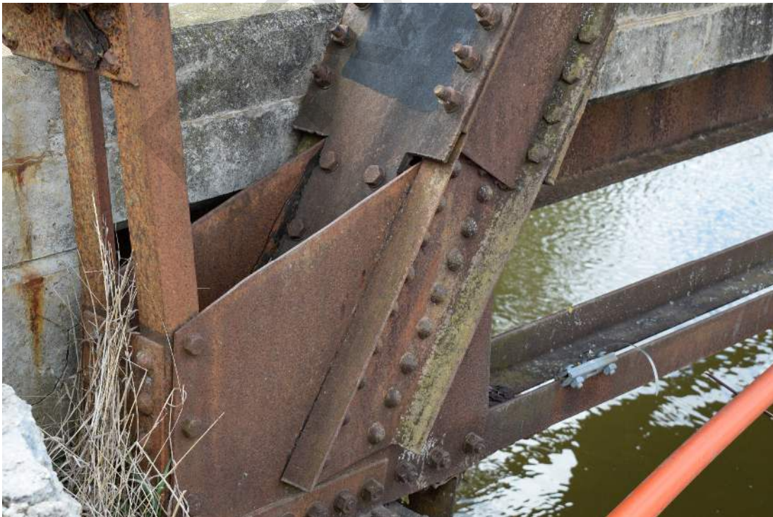
Figure 50: Example of past repair as seen on northwest corner of bridge
