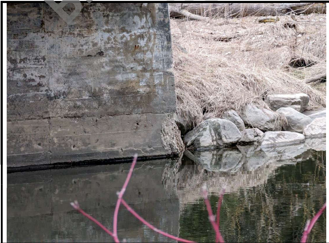
Photo 22 Concrete disintegration observed east abutment and at the interface of the southeast wingwall
