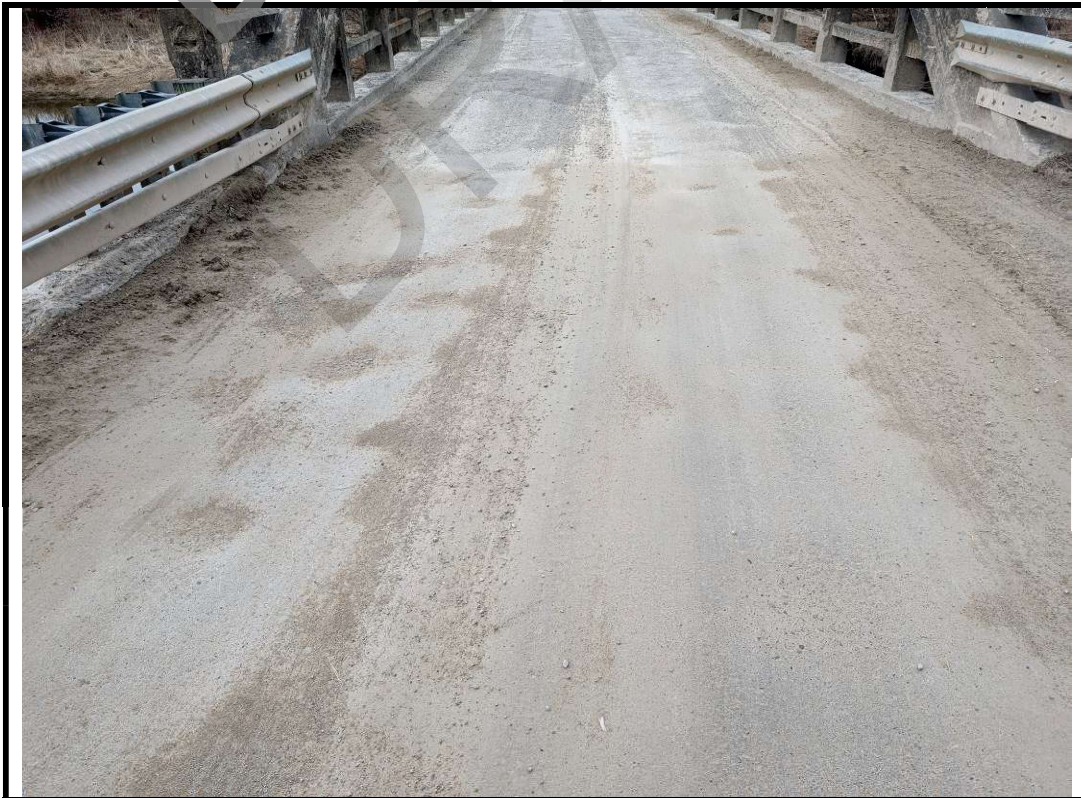
Photo 8 Potholes on west approach near deck
