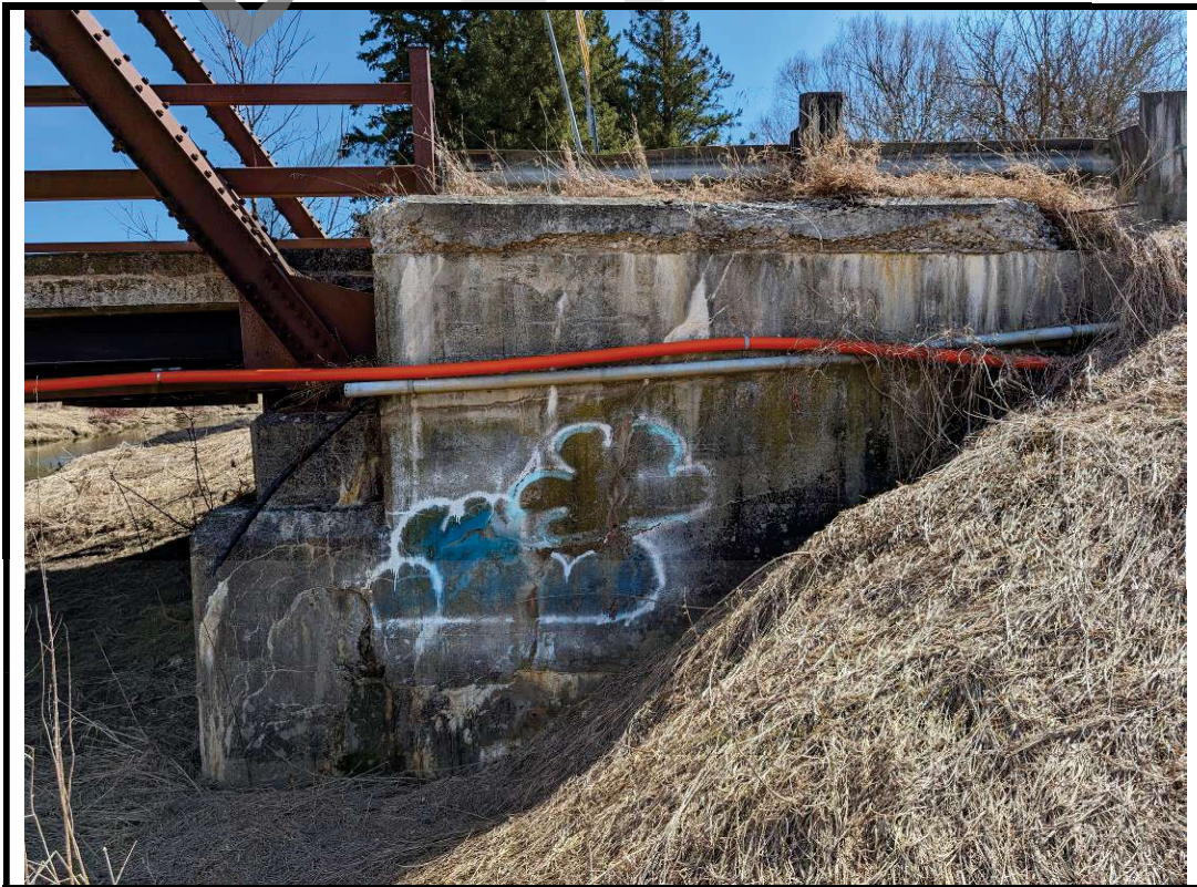
Photo 18 Cracks with efflorescence and graffiti at northeast wing wall
