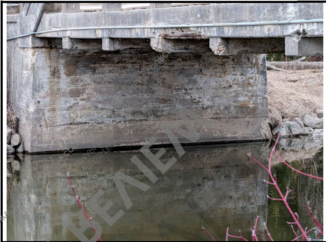
Photo 15 Scaling on foundation of east abutment wall
