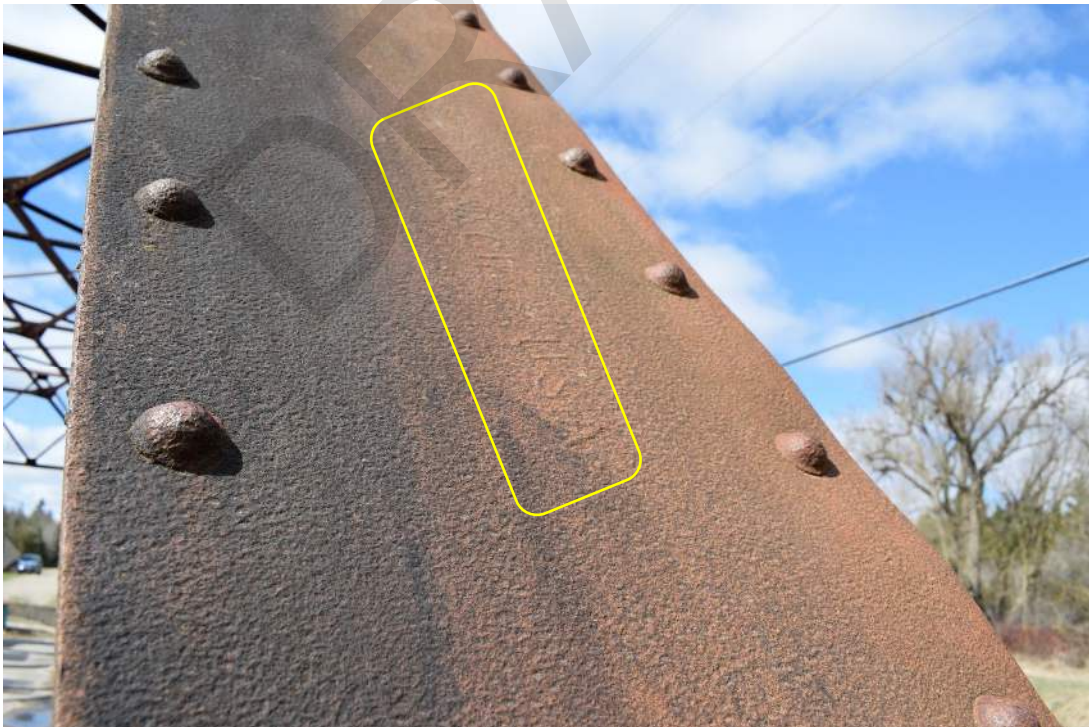
Figure 54 Maker's mark identifying original steel to be a product of 'Carnegie USA'
