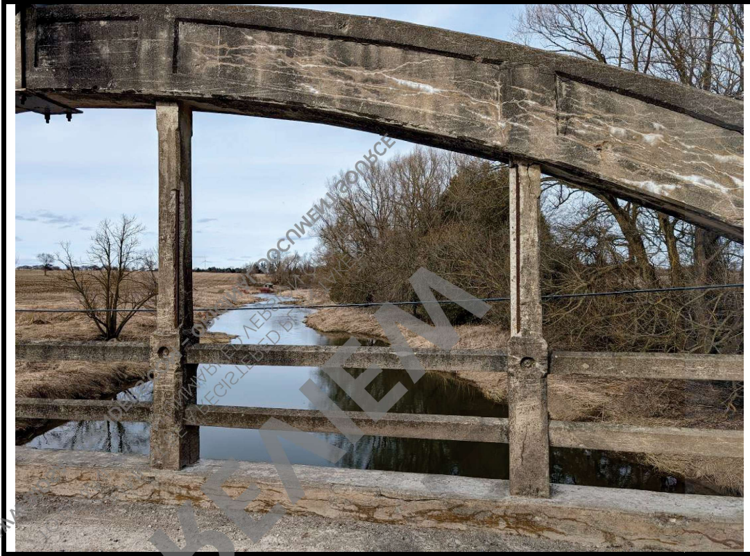
Photo 11 Spall with exposed corroded reinforcement on east truss vertical.
