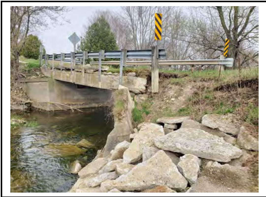
Photo 12 Northwest wingwall collapse and disconnected from abutment
