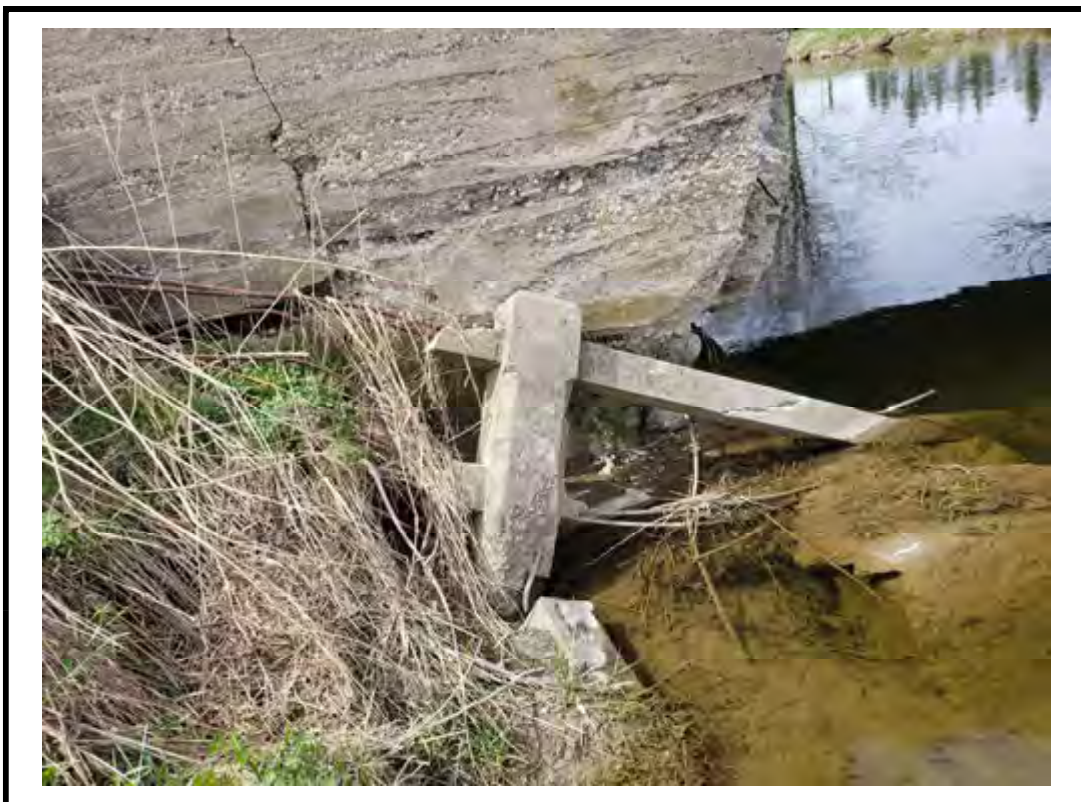
Photo 8 Bridge barrier broken / detached
