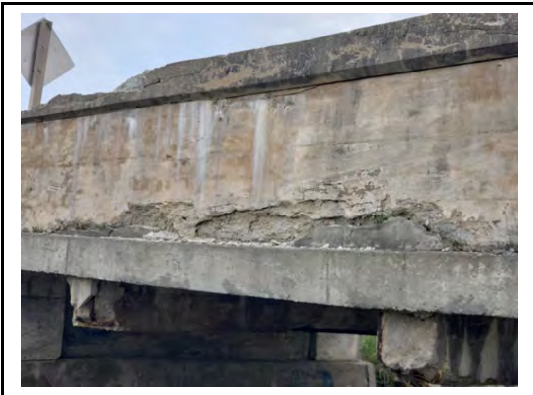
Photo 10 Spalls with exposed corroded reinforcement on north end of floor beam
