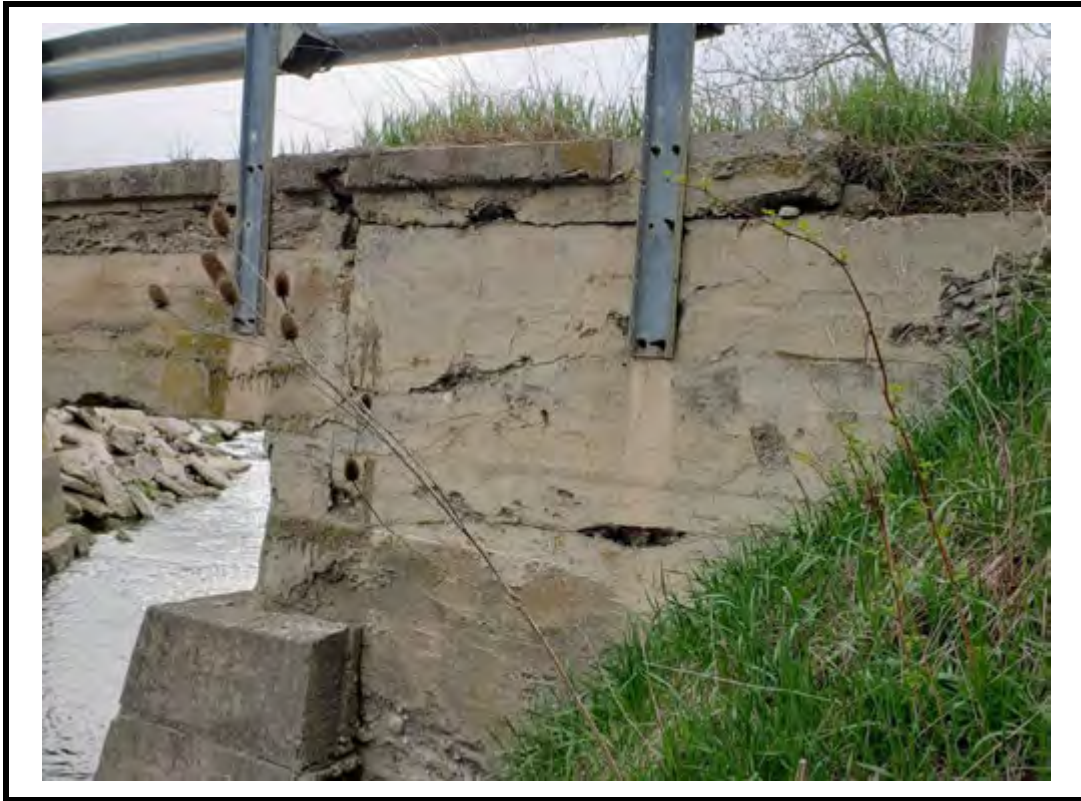
Photo 13 Wide cracks, and spalls on SE wingwall
