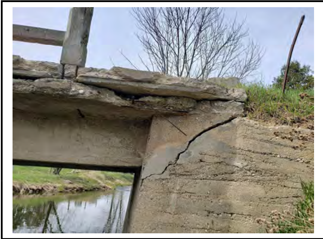
Photo 9 Large crack noted on wing wall
