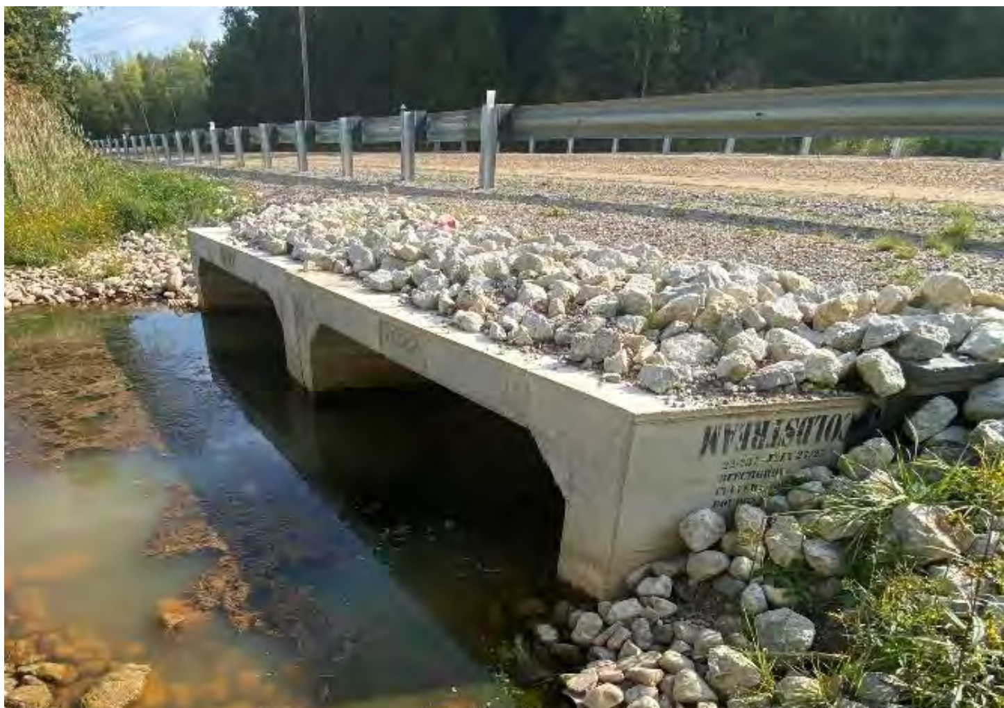
Precast Concrete Box Culverts
