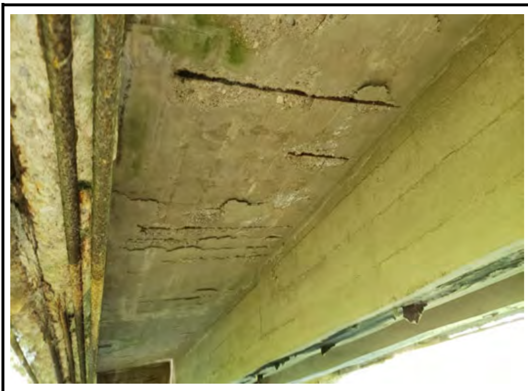
Photo 8 Large spalls with exposed corroded reinforcement on soffit and girder
