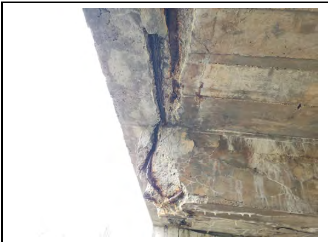
Photo 14 Spall with exposed corroded reinforcement at edge of concrete deck.
