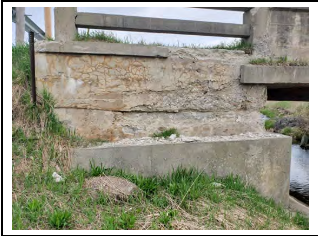
Photo 11 Spalls and stained cracks on NE wingwall
