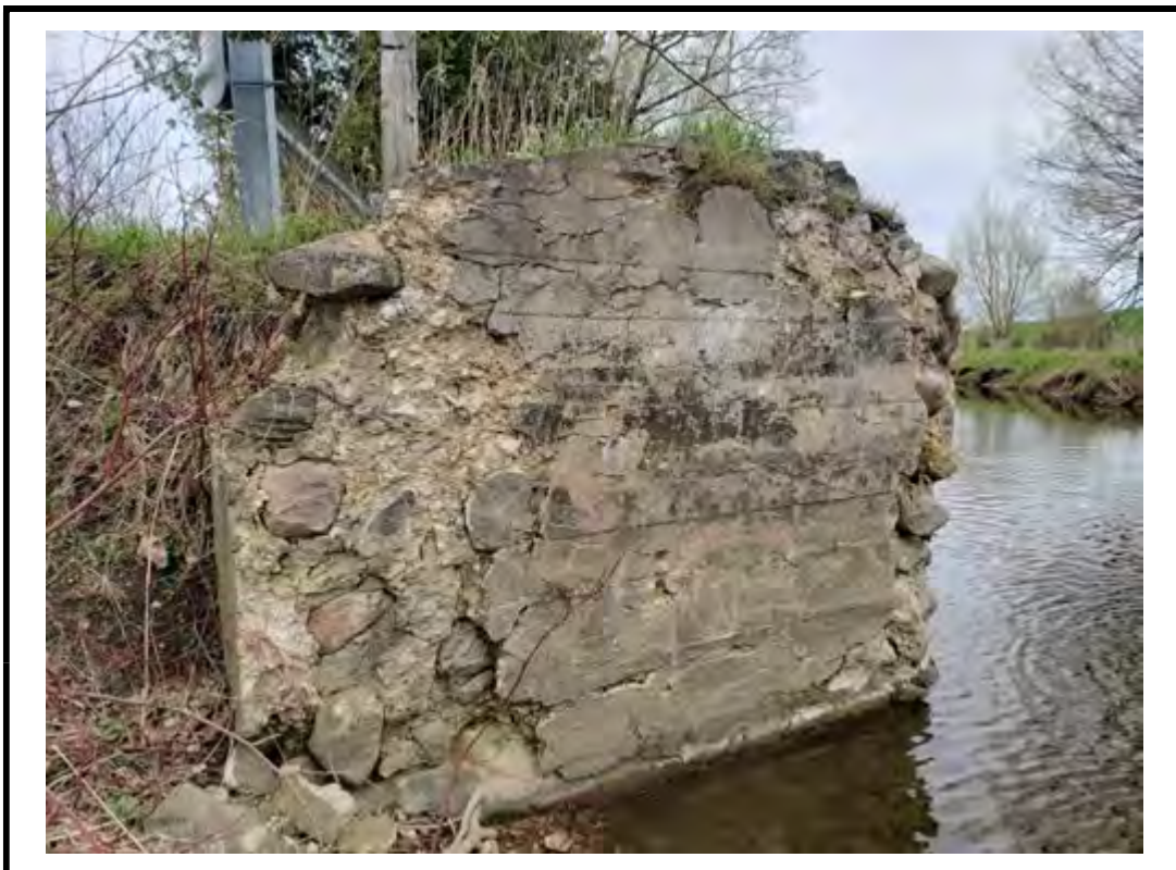
Photo 6 Large spalls and severe concrete disintegration noted on northeast wingwall
