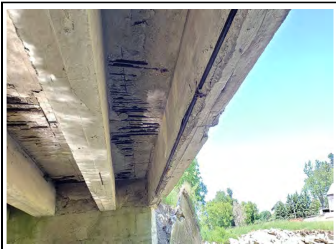
Photo 10 Spall with exposed corroded reinforcement on south exterior girder
