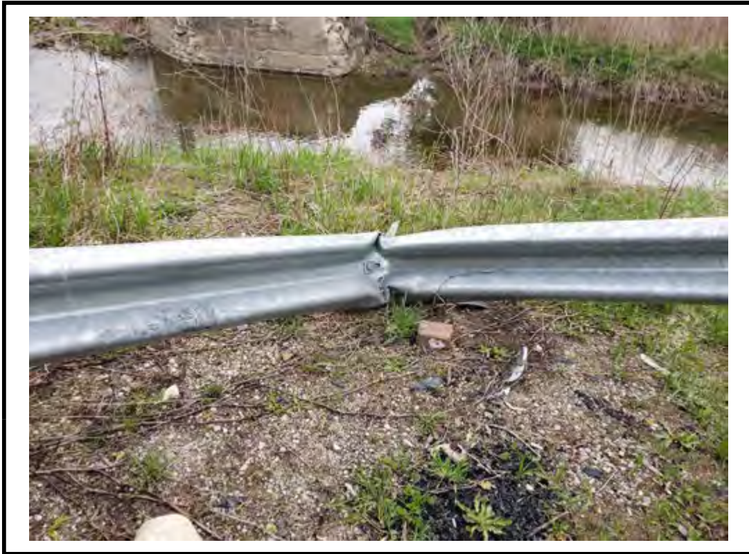
Photo 5 Damaged/ broken steel beam rail at west approach
