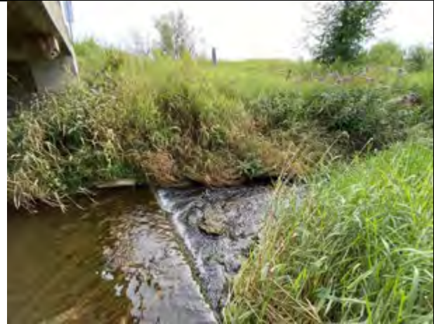
Photo: 12 Culvert outlet is perched at outlet. Facing east.
