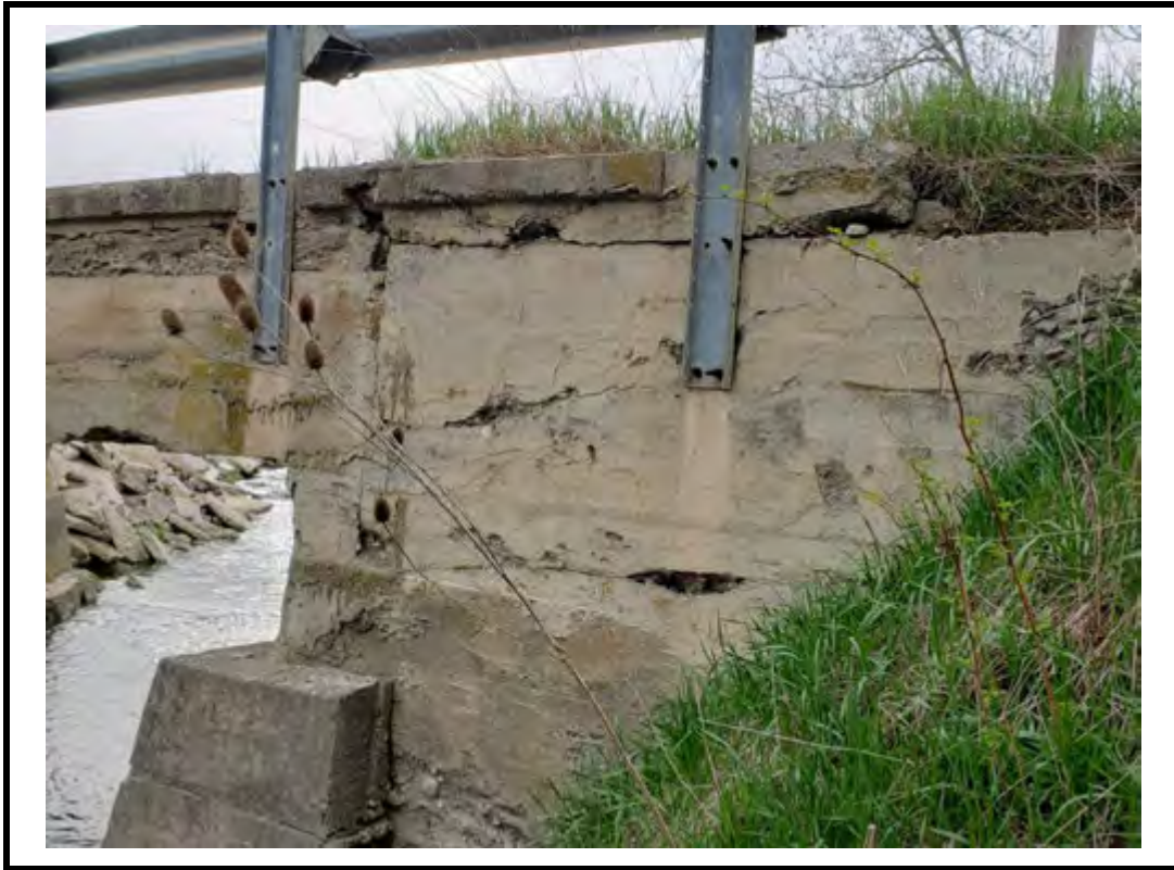
Photo 13 Wide cracks, and spalls on SE wingwall
