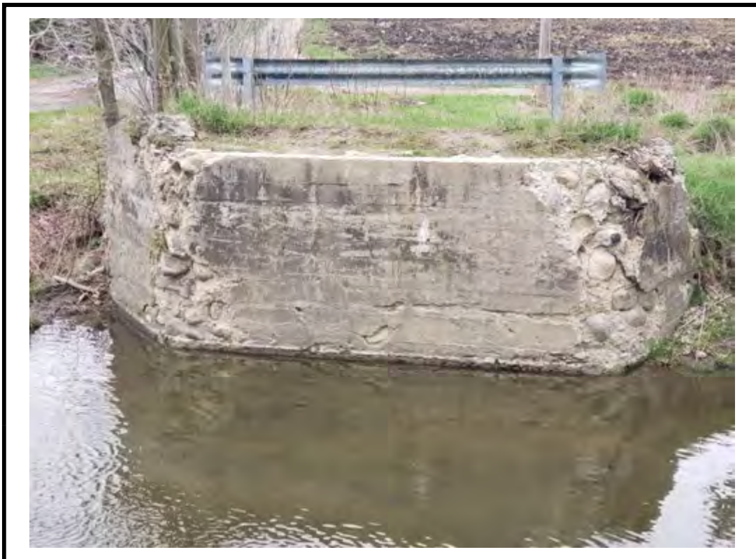
Photo 4 Large spalls, scaling and concrete disintegration noted on west abutment wall
