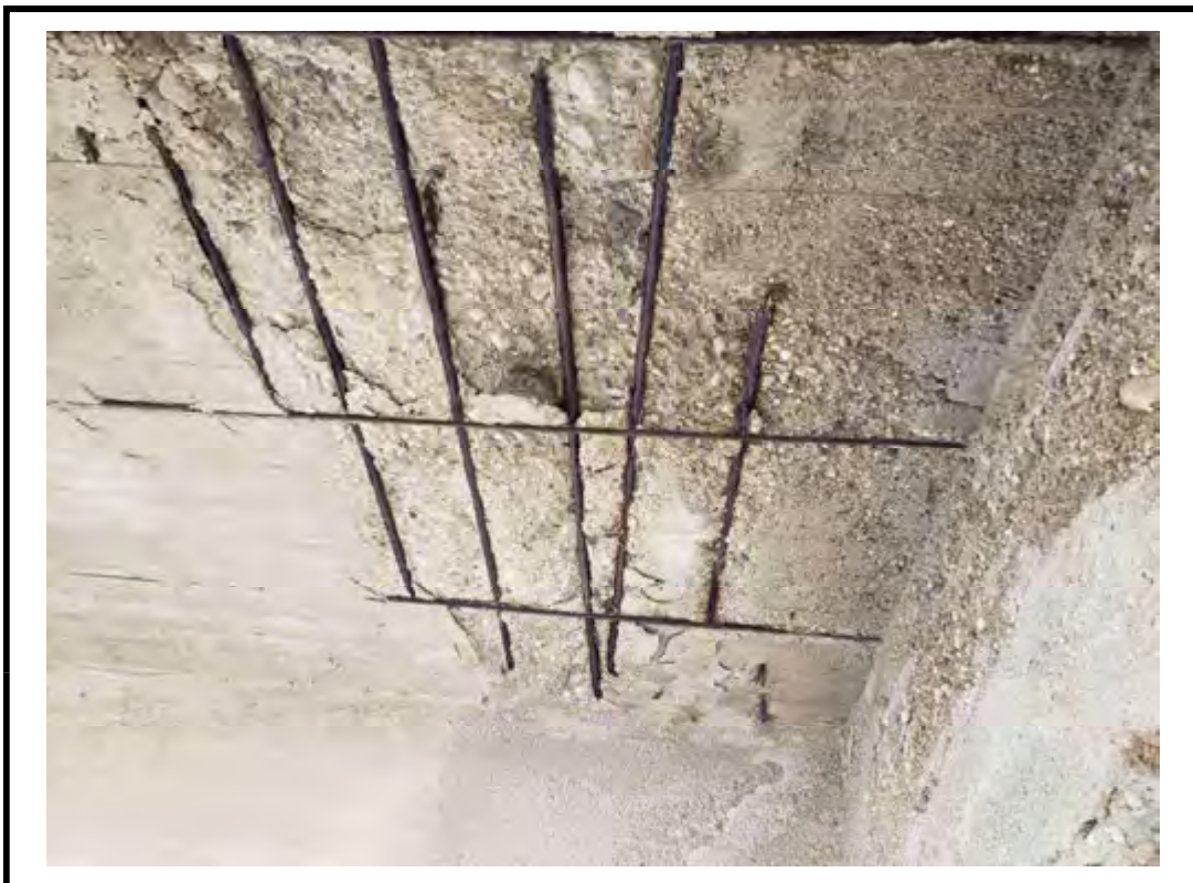
Photo 12 Exposed Corroded Reinforcement
