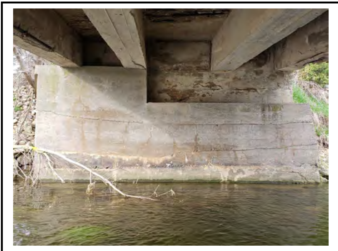
Photo 14 Localized cracks with staining at abutments.
