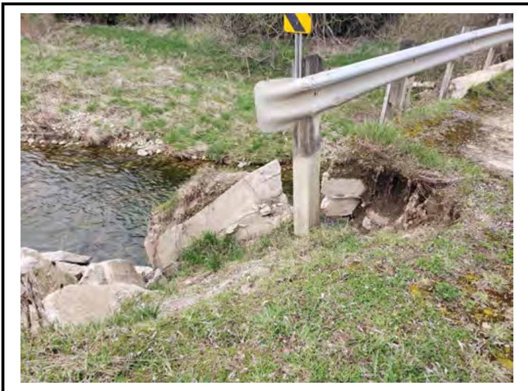
Photo 8 Spalls in concrete around barrier posts
