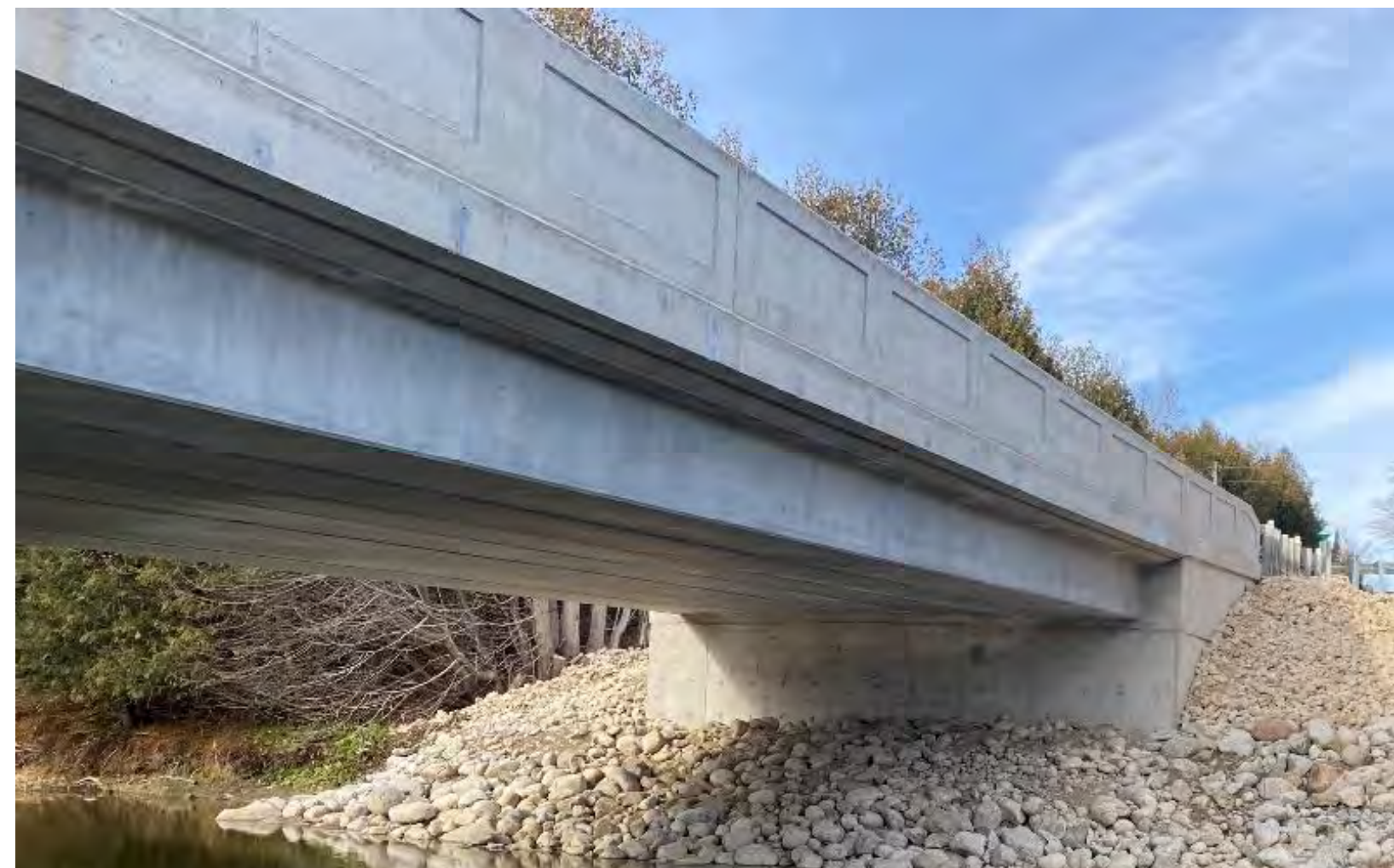
Prestressed Concrete Box Girders
