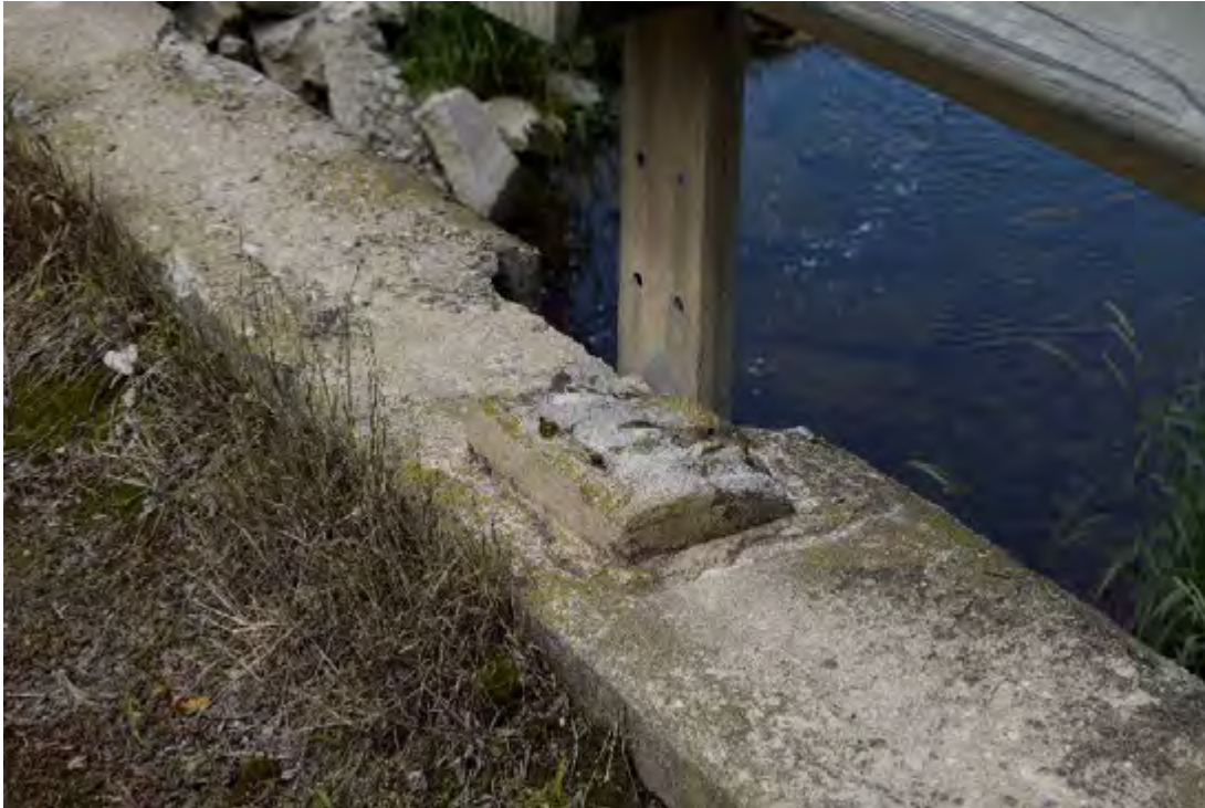
FIGURE 19: REMAINS OF ORIGINAL CAST GUARD RAIL
