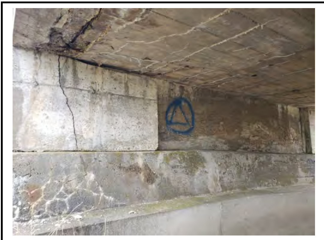
Photo 12 Cracks and stains on east abutment wall
