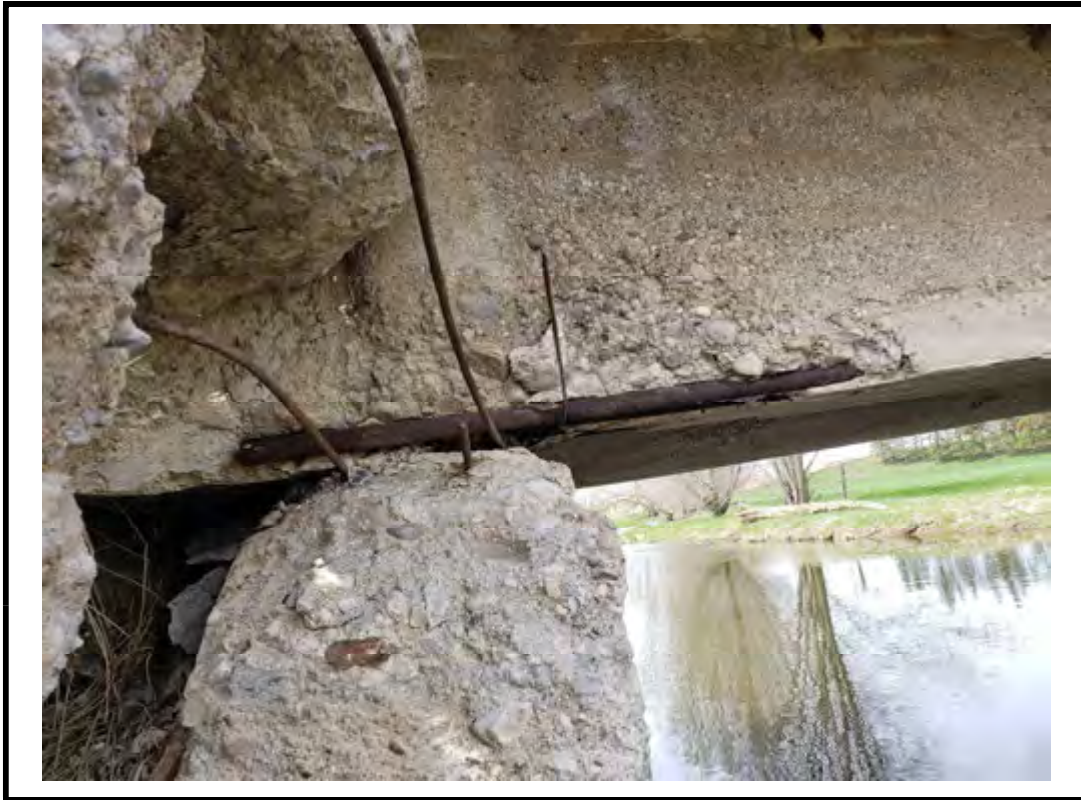
Photo 12 Exposed Corroded Reinforcement
