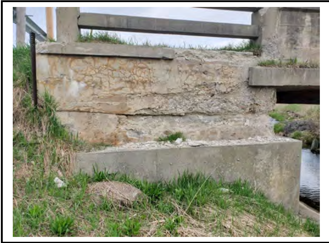
Photo 11 Spalls and stained cracks on NE wingwall
