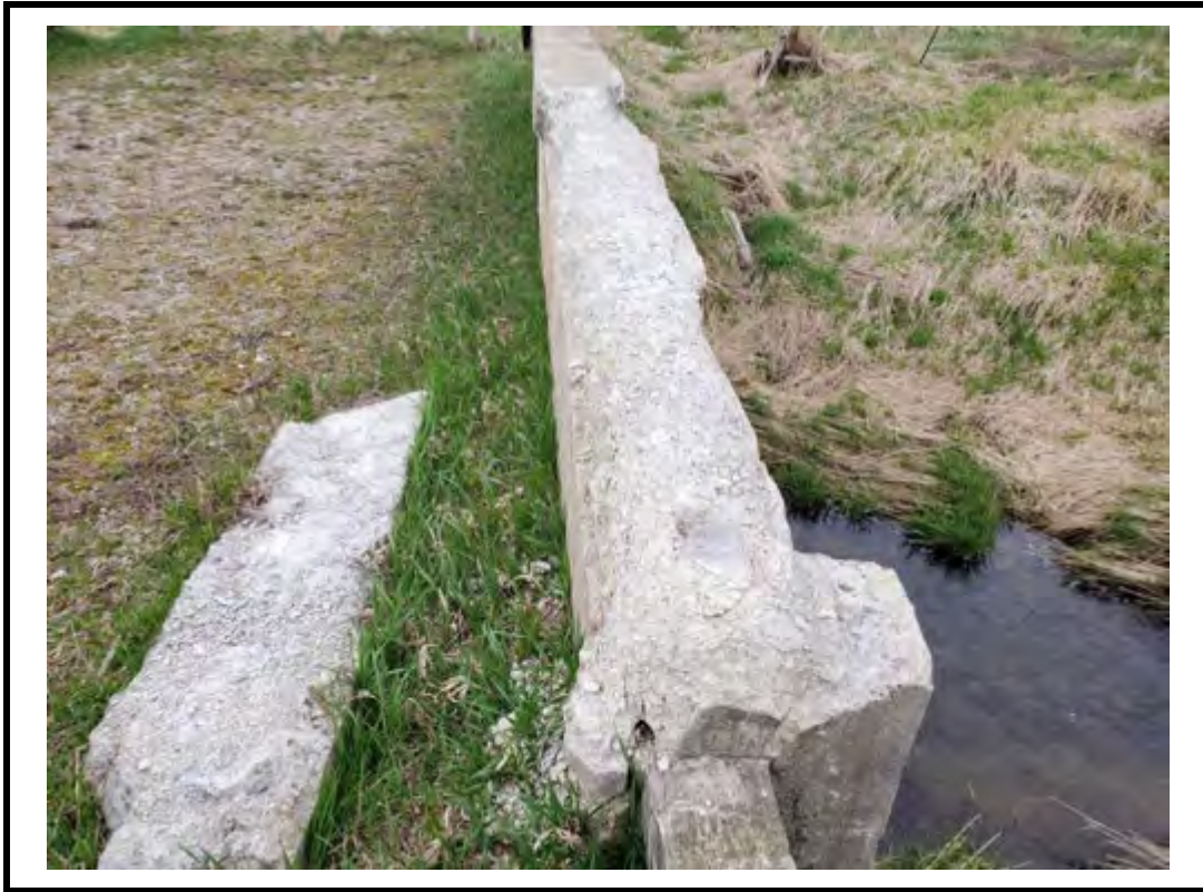
Photo 7 Concrete disintegration on north deck barrier
