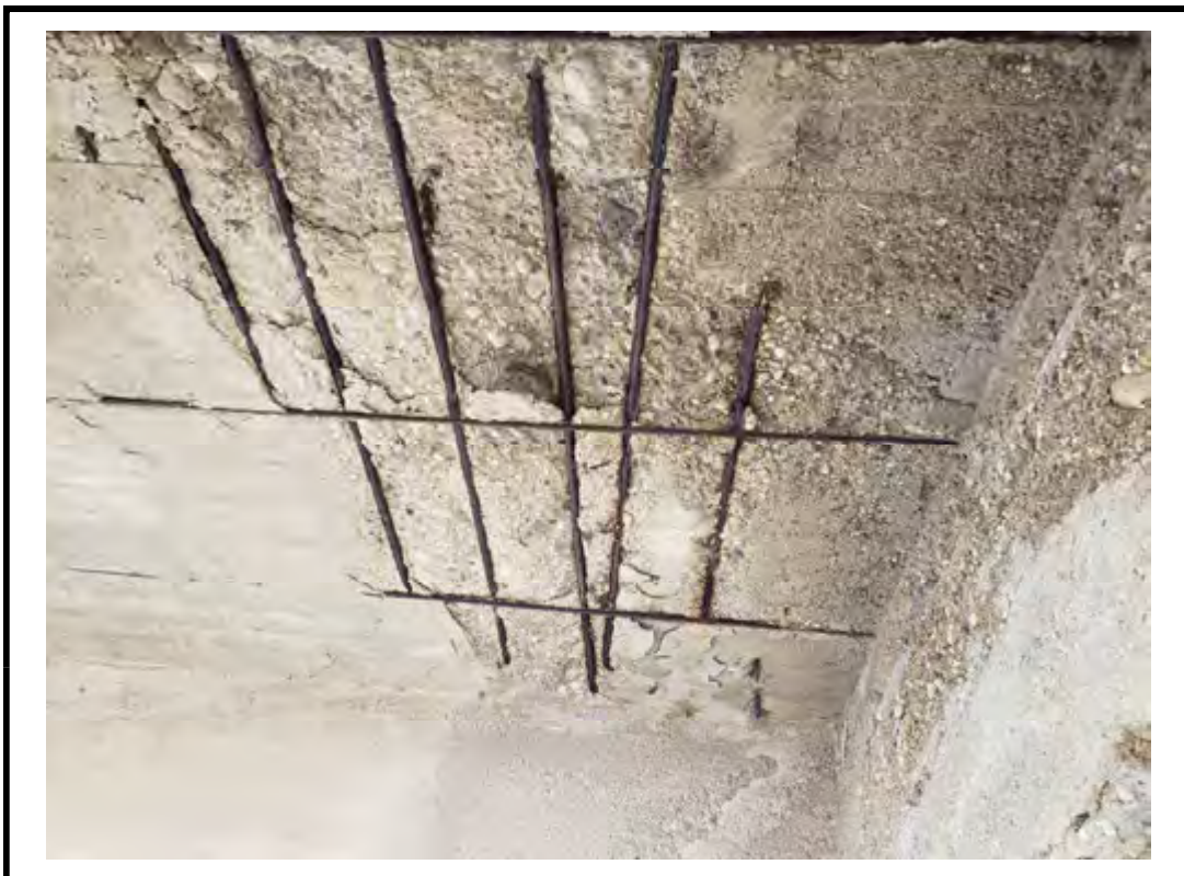
Photo 12 Exposed Corroded Reinforcement
