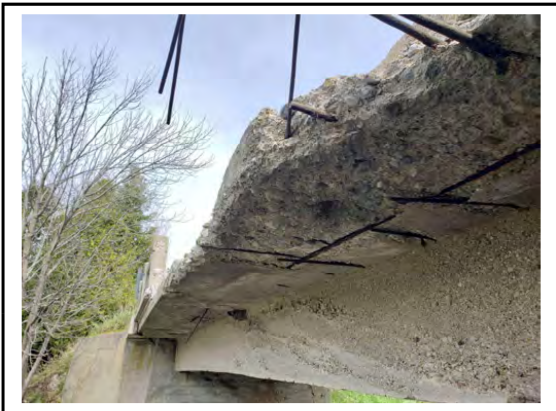
Photo 14 Large Spall with Exposed Corroded Reinforcement on the Exterior Face
