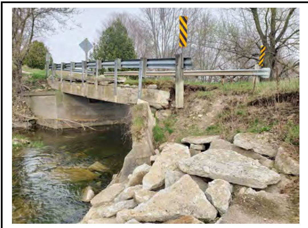
Photo 12 Northwest wingwall collapse and disconnected from abutment
