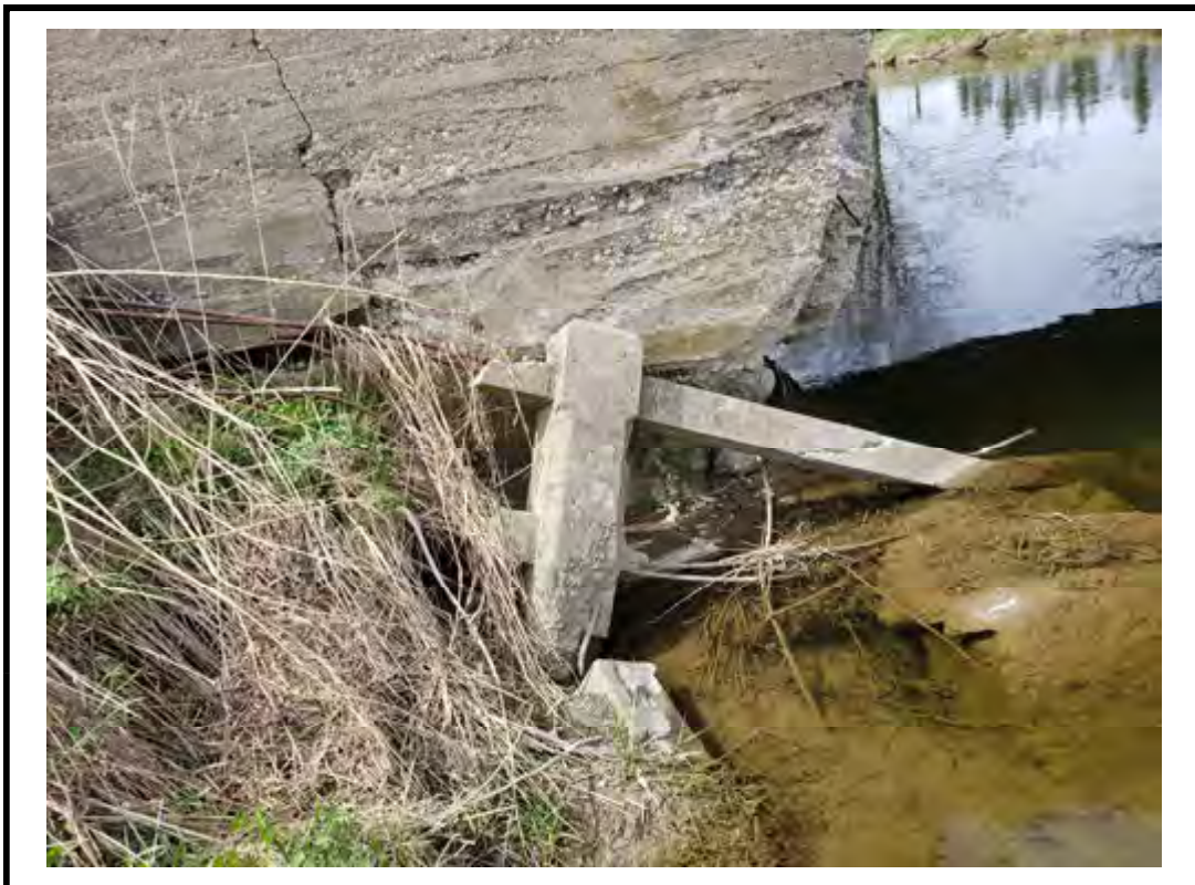
Photo 8 Bridge barrier broken / detached
