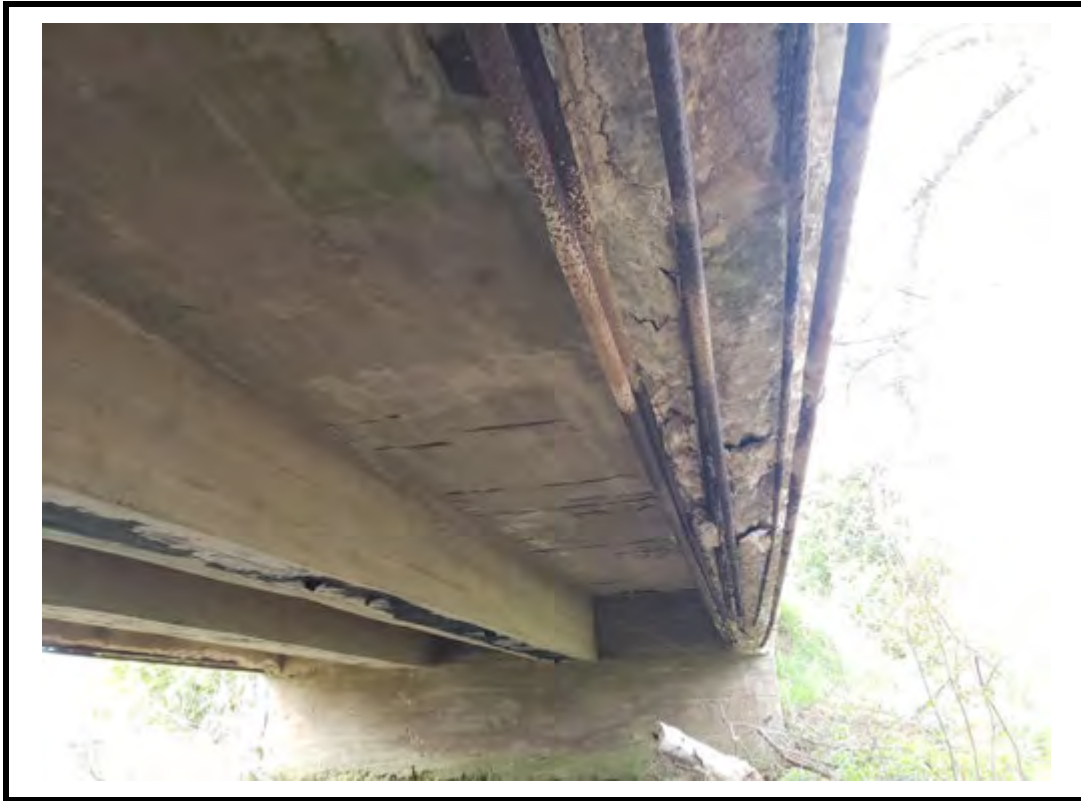
Photo 9 Large spall with exposed corroded reinforcement on underside of exterior girder
