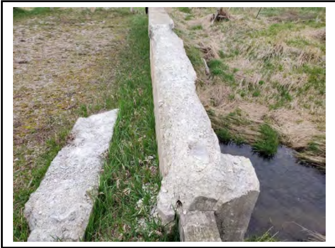
Photo 7 Concrete disintegration on north deck barrier
