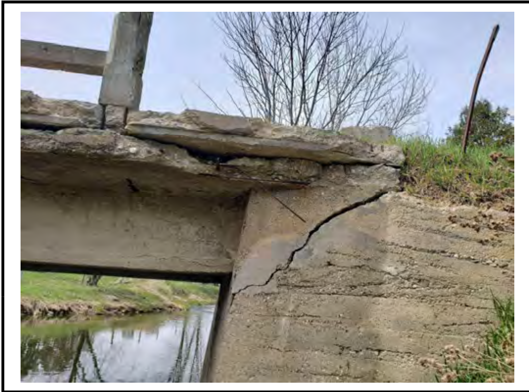
Photo 9 Large crack noted on wing wall
