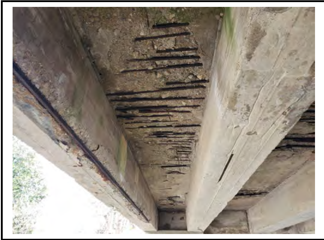
Photo 9 Spalls and delaminations with exposed corroded reinforcement on east deck soffit
