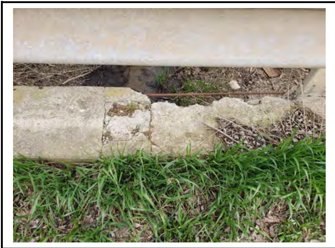
Photo 7 Large spalls with exposed corroded reinforcement noted on curbs
