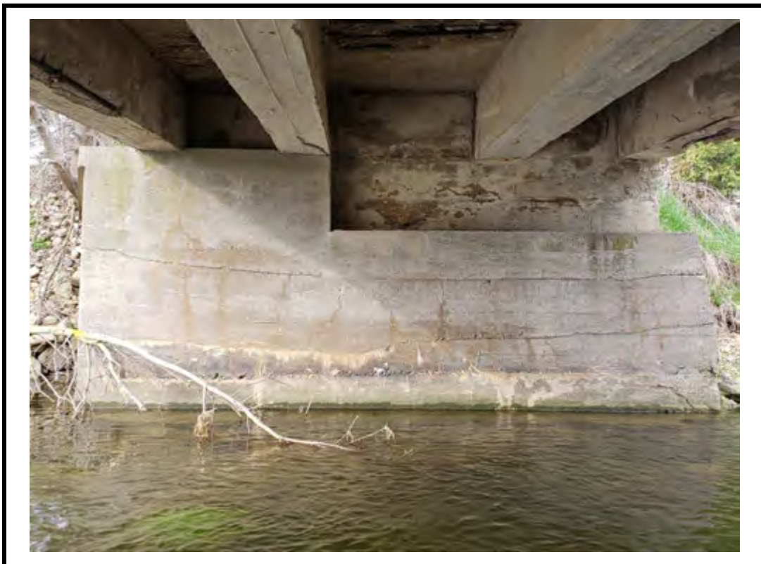
Photo 14 Localized cracks with staining at abutments.
