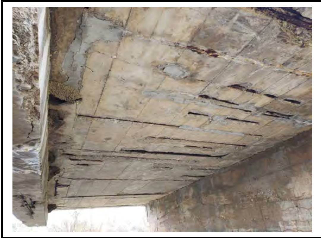
Photo 9 Spalls with exposed corroded reinforcement and efflorescence on north soffit
