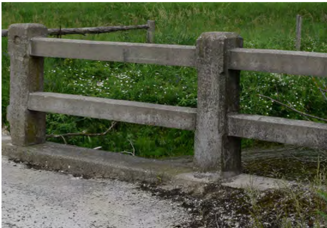
FIGURE 4: CLOSEUP OF REMAINING RAILING SHOWING CAST DETAILS
