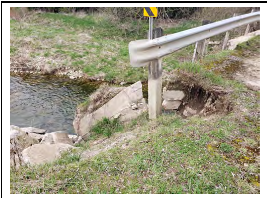
Photo 8 Spalls in concrete around barrier posts
