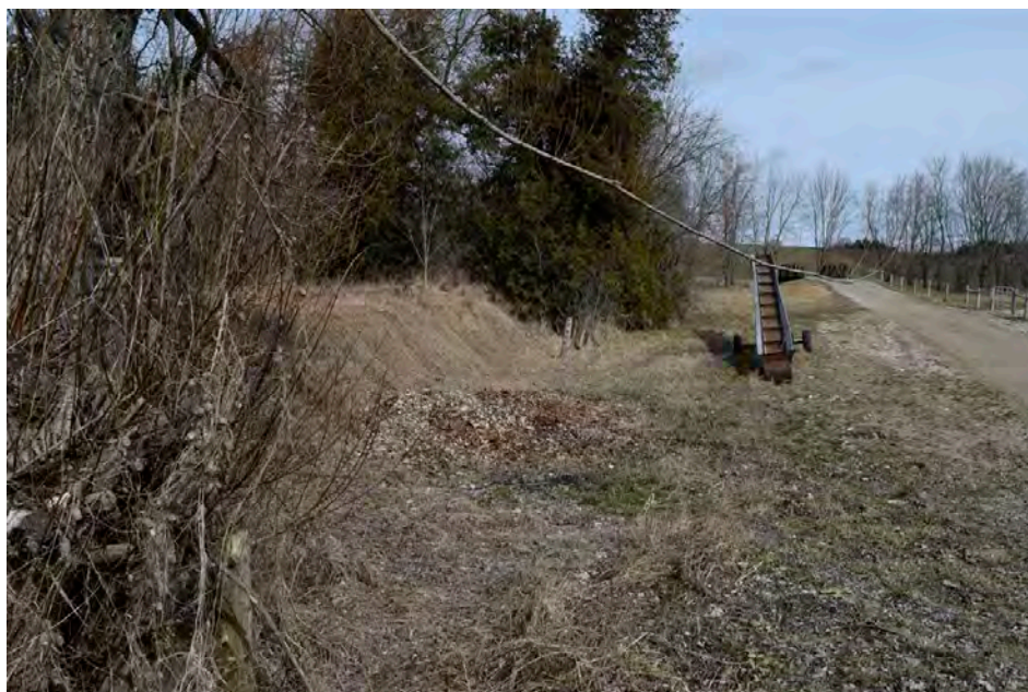
IMAGE 12: VIEW OF 32-P WITH STEEP, OVERGROWN DITCHES TO POORLY DRAINED AREA, FACING NORTH
