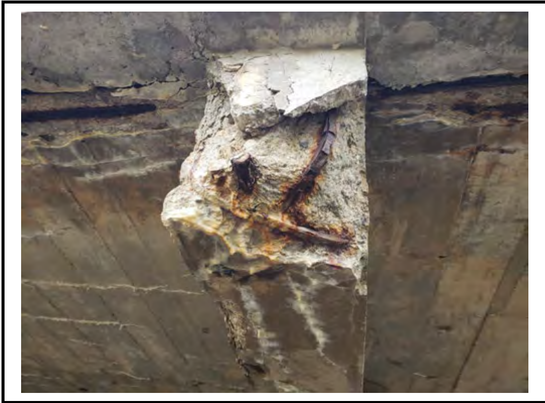
Photo 13 Large spall with exposed corroded reinforcement at concrete beams.
