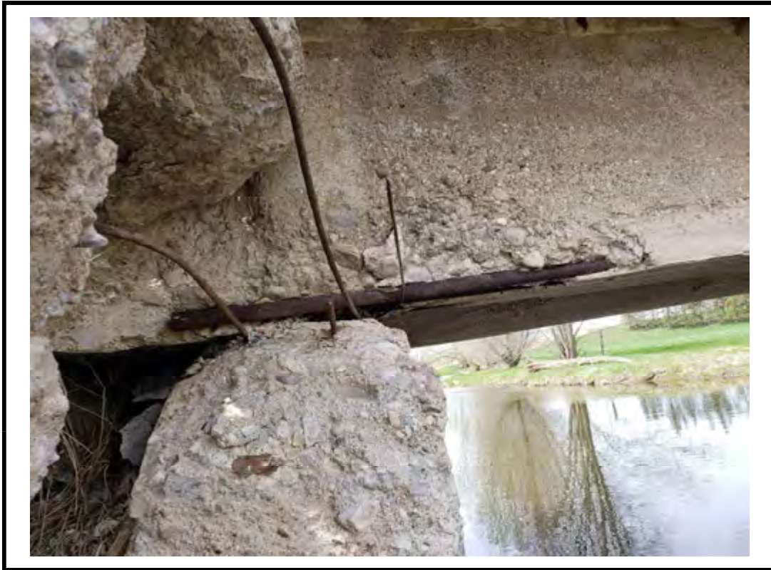
Photo 12 Exposed Corroded Reinforcement
