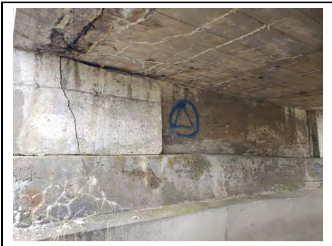
Photo 12 Cracks and stains on east abutment wall
