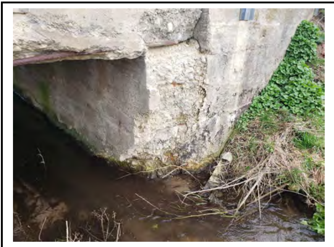
Photo 10 Severe scaling and spalls observed on southwest wingwall
