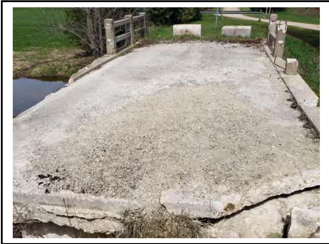
Photo 7 Moderate scaling and large spalls on concrete deck
