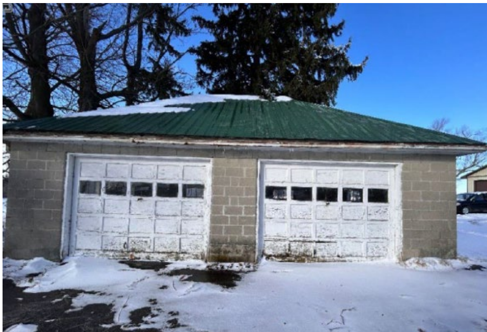
PHOTO 8: Concrete Block Garage (MHBC 2025)
