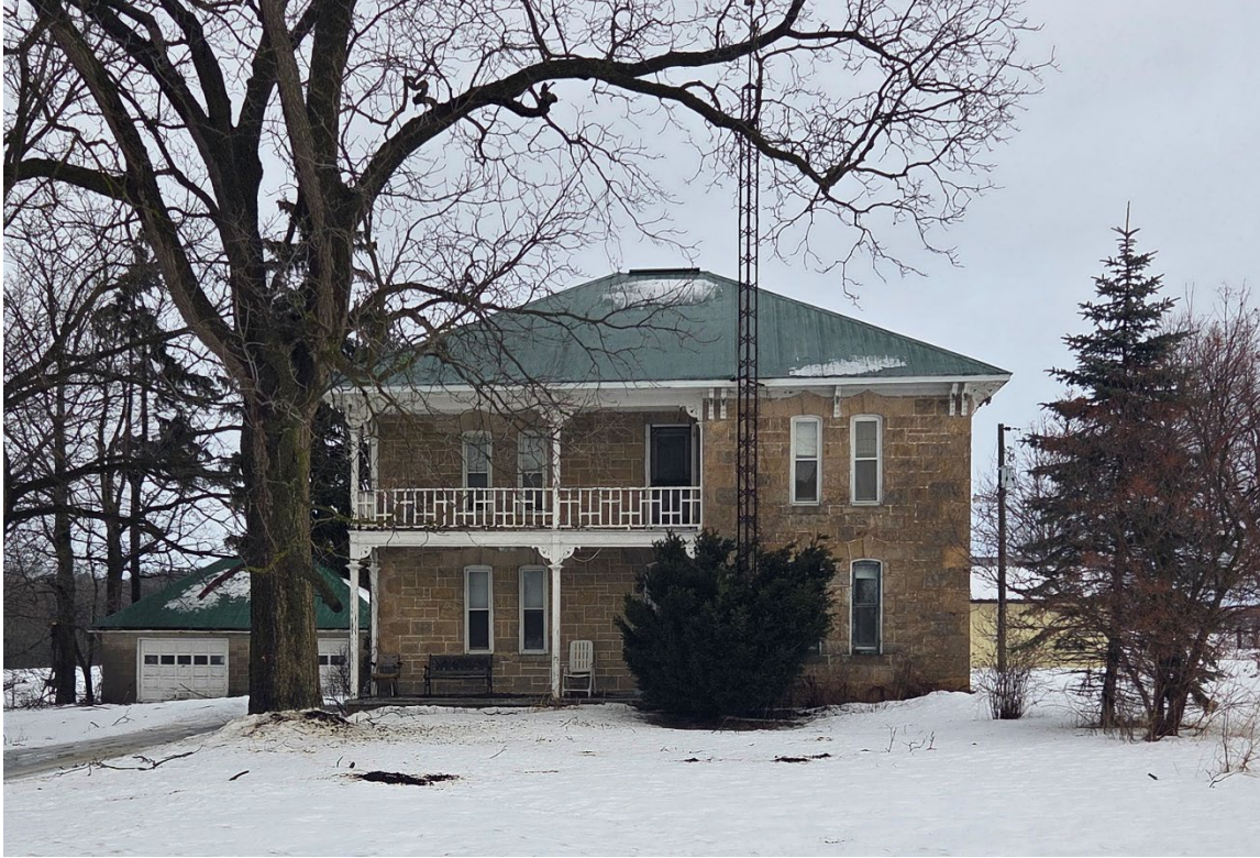
PHOTO 1: 2-Storey Dwelling Front (South) Elevation (Township 2026)
