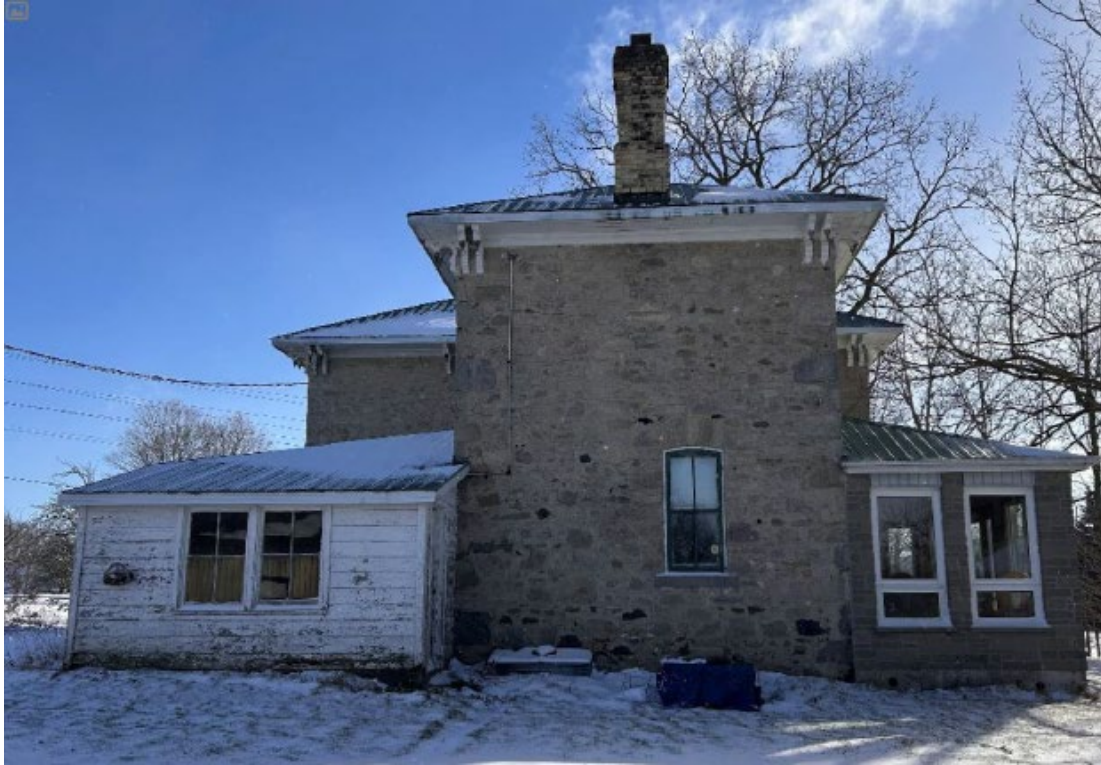
PHOTO 5: 2-Storey Dwelling Rear (North) Elevation (MHBC 2025)
