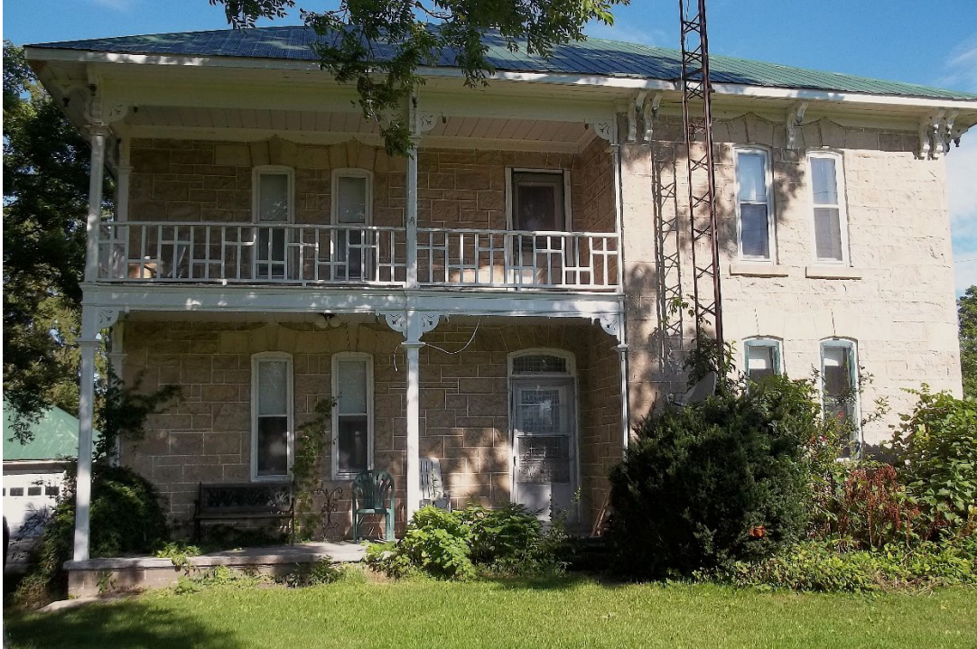
PHOTO 2: 2-Storey Dwelling Front (South) Elevation (Township 2017)
