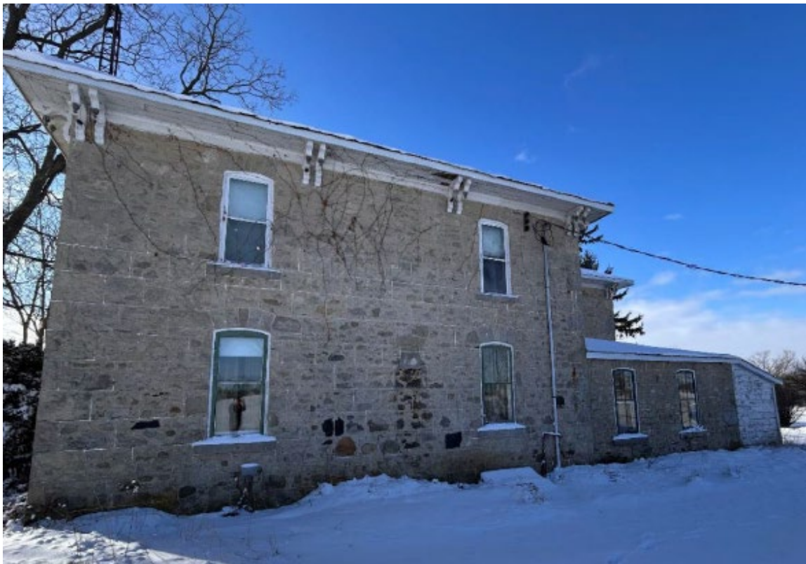
PHOTO 4: 2-Storey Dwelling Side (East) Elevation (MHBC 2025)
