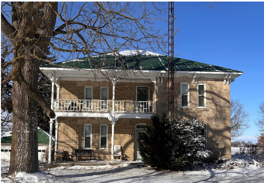
Figure 6 – front façade (south elevation)
