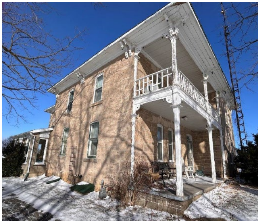
PHOTO 6: 2-Storey Dwelling Side (West) Elevation (MHBC 2025)
