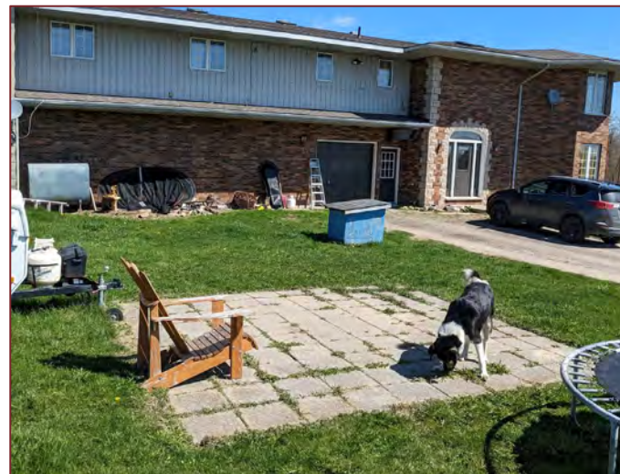
Photo 2: View of an out of use heating oil AST located on the southwest corner of the house.
