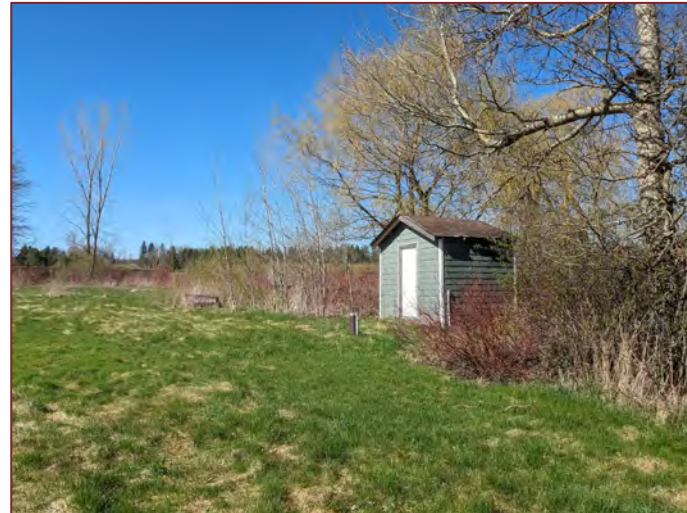
Photo 16: View of the pumphouse located on the north portion of the Site.
