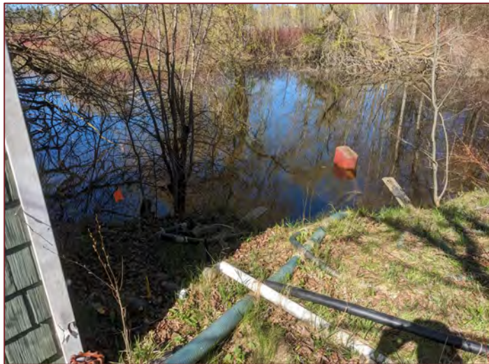
Photo 17: View the north most pond on the Site (near pumphouse).
