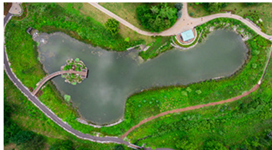
Fig.8: Stormwater management pond with passive recreational uses (Source: City of Richmond Hill)
