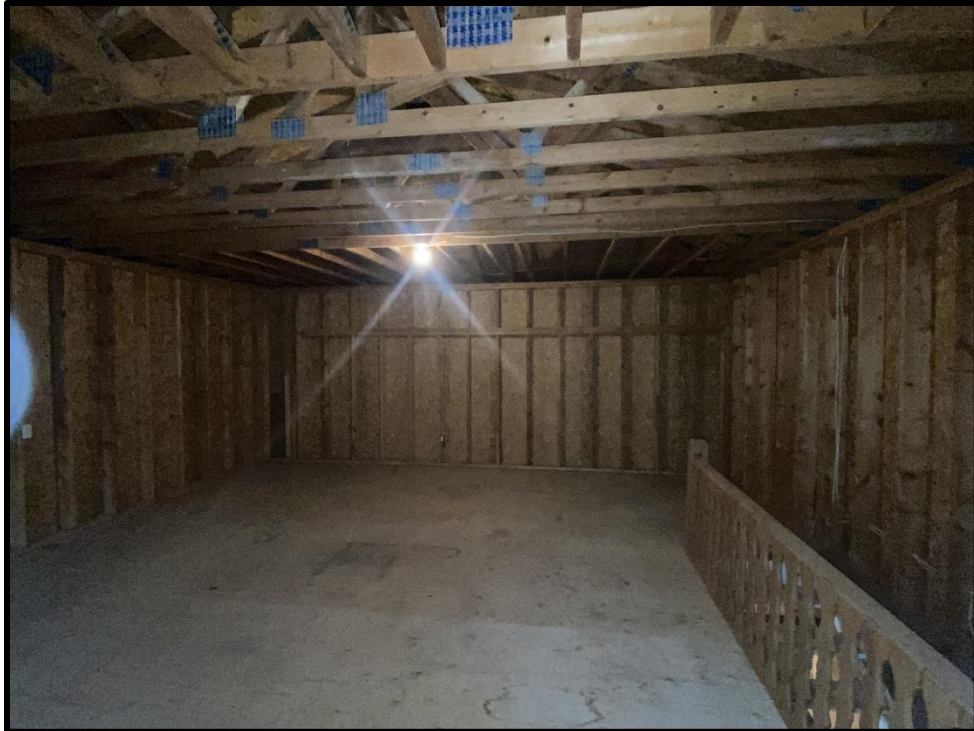
Image 79: Garage Interior – Unfinished Walls and Plywood Floor of Garage Loft (Photograph taken August 28, 2025)
