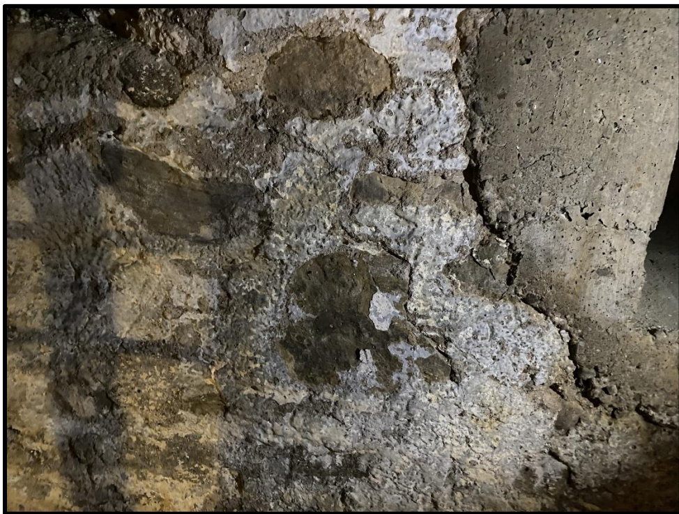
Image 64: Residence Interior – Parged Stone and Brick Basement Walls (Photograph taken August 28, 2025)
