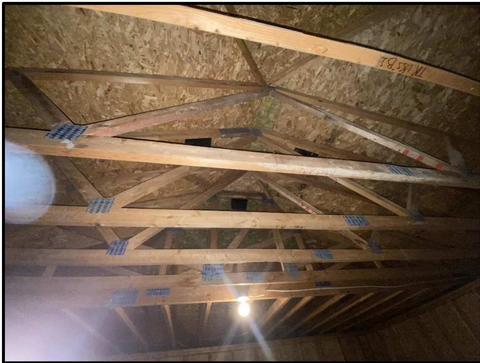
Image 78: Garage Interior – Rafters and Joists of Open Roof in Garage (Photograph taken August 28, 2025)
