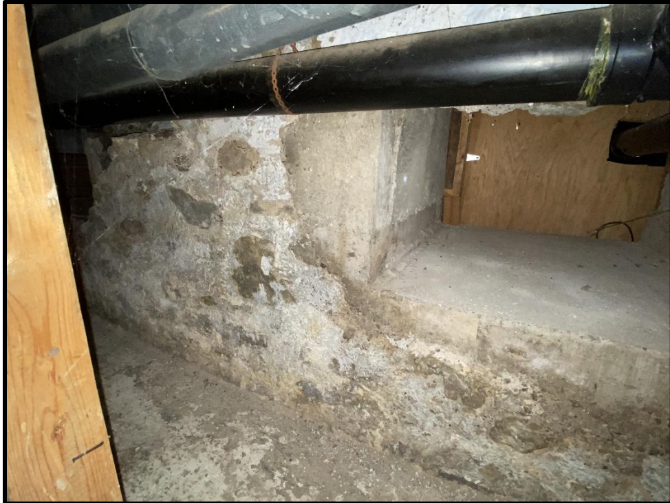
Image 65: Residence Interior – Stone and Parging on Basement Walls (Photograph taken August 28, 2025)
